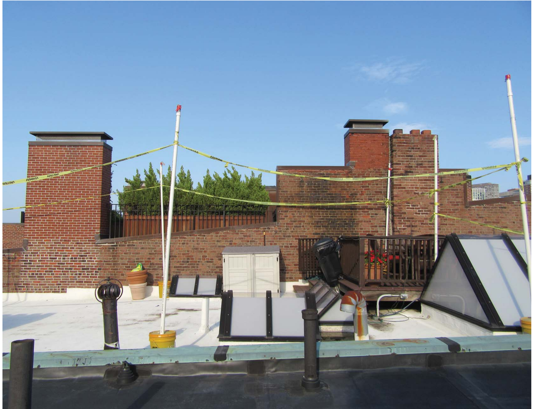
Mock-Up Looking East
