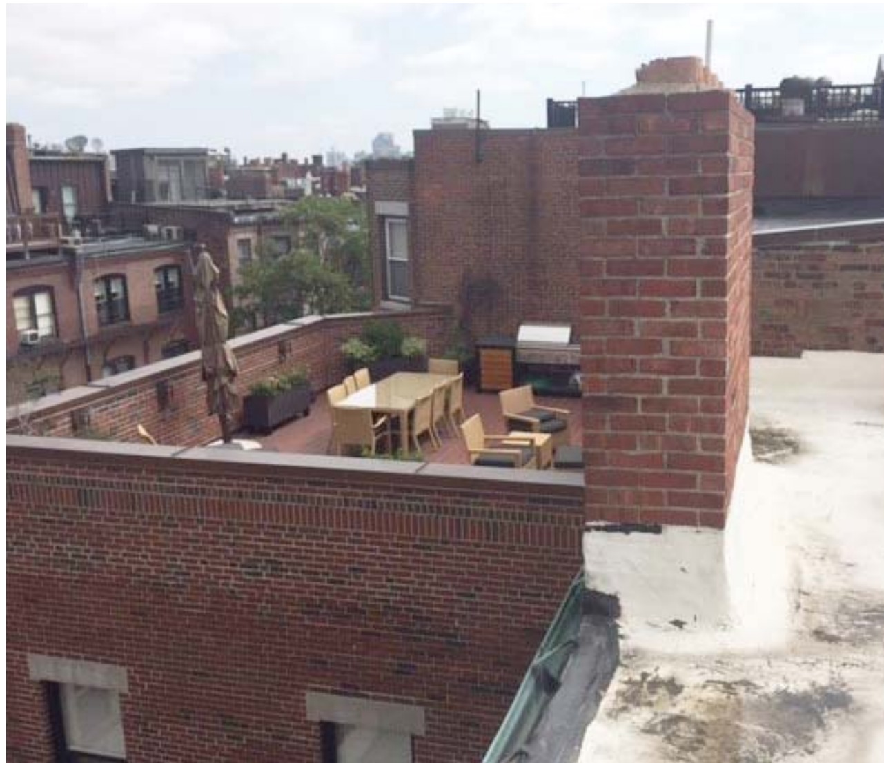
Existing Roof Decks & Penthouses Looking East
