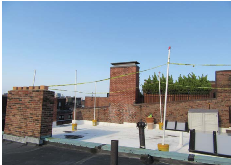
Mock-Up Looking West
