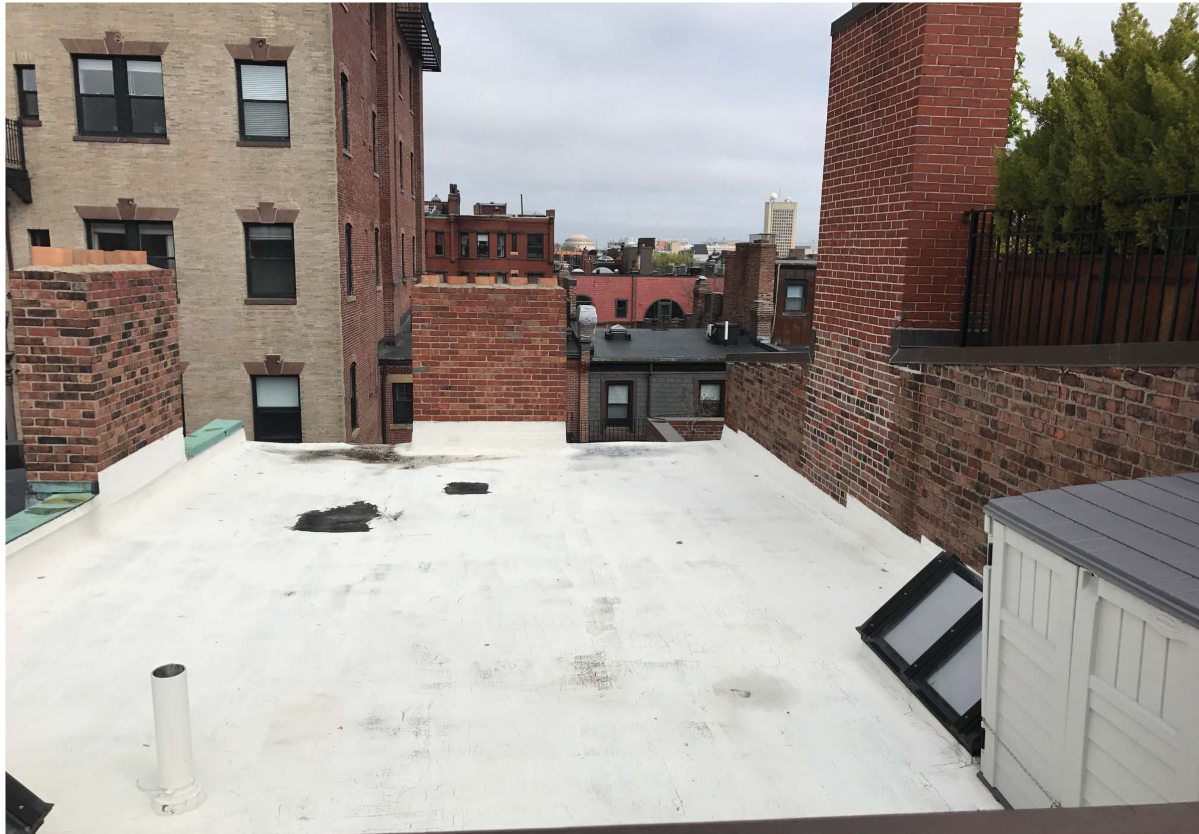
Existing Roof Looking North
