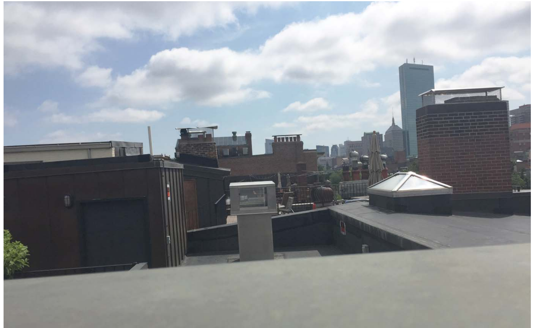
Existing Roof Decks & Penthouses Looking East
