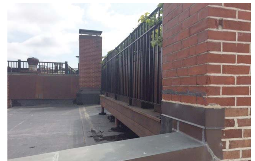
Existing Roof Decks & Penthouses Looking East
