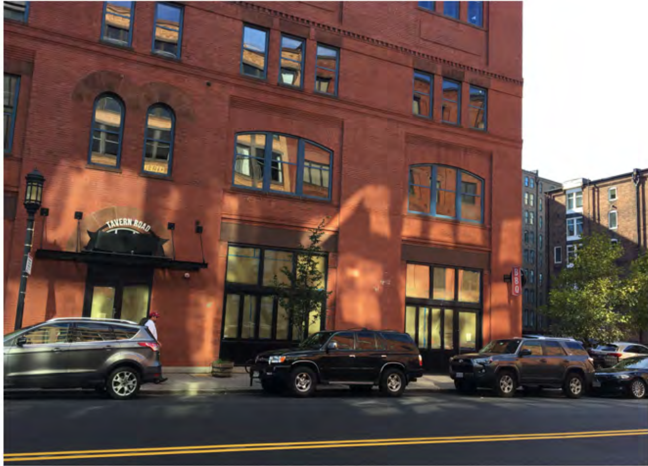
VIEW FROM FARNSWORTH STREET
