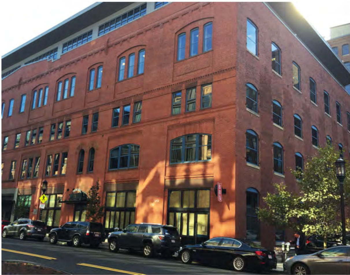
CLOSE UP VIEW FROM ACROSS THE STREET
