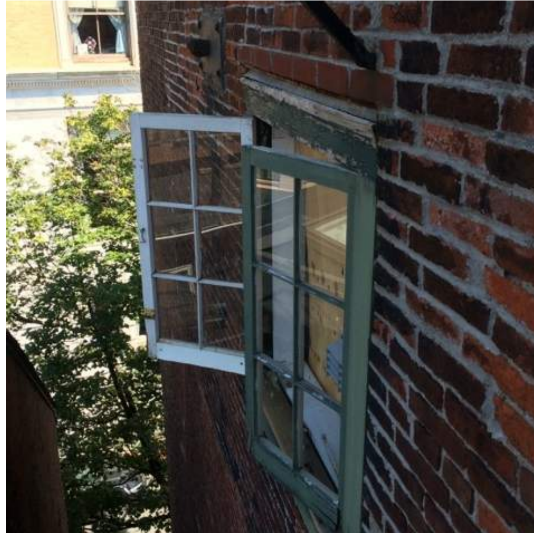
SIDE ALLEY EXISTING CONDITIONS
