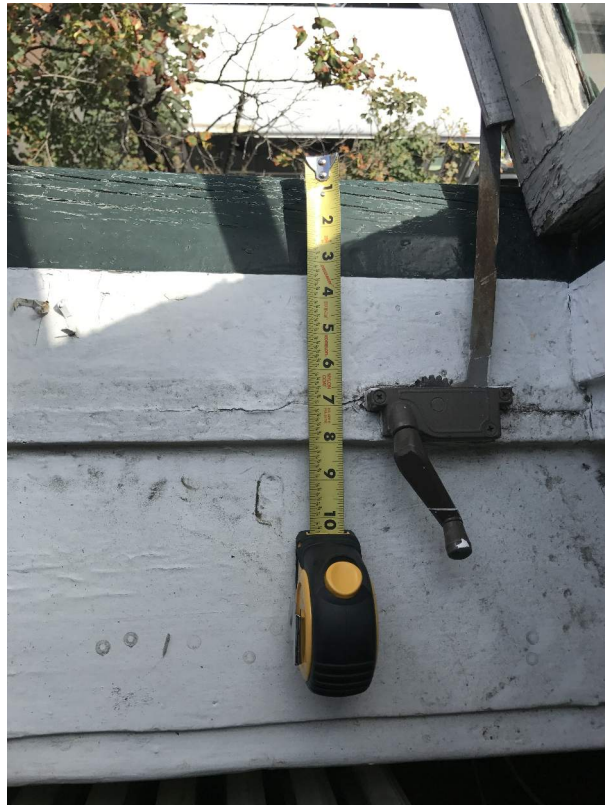
TYPICAL EXISTING CASEMENT WOOD WINDOW, SINGLE PANE
