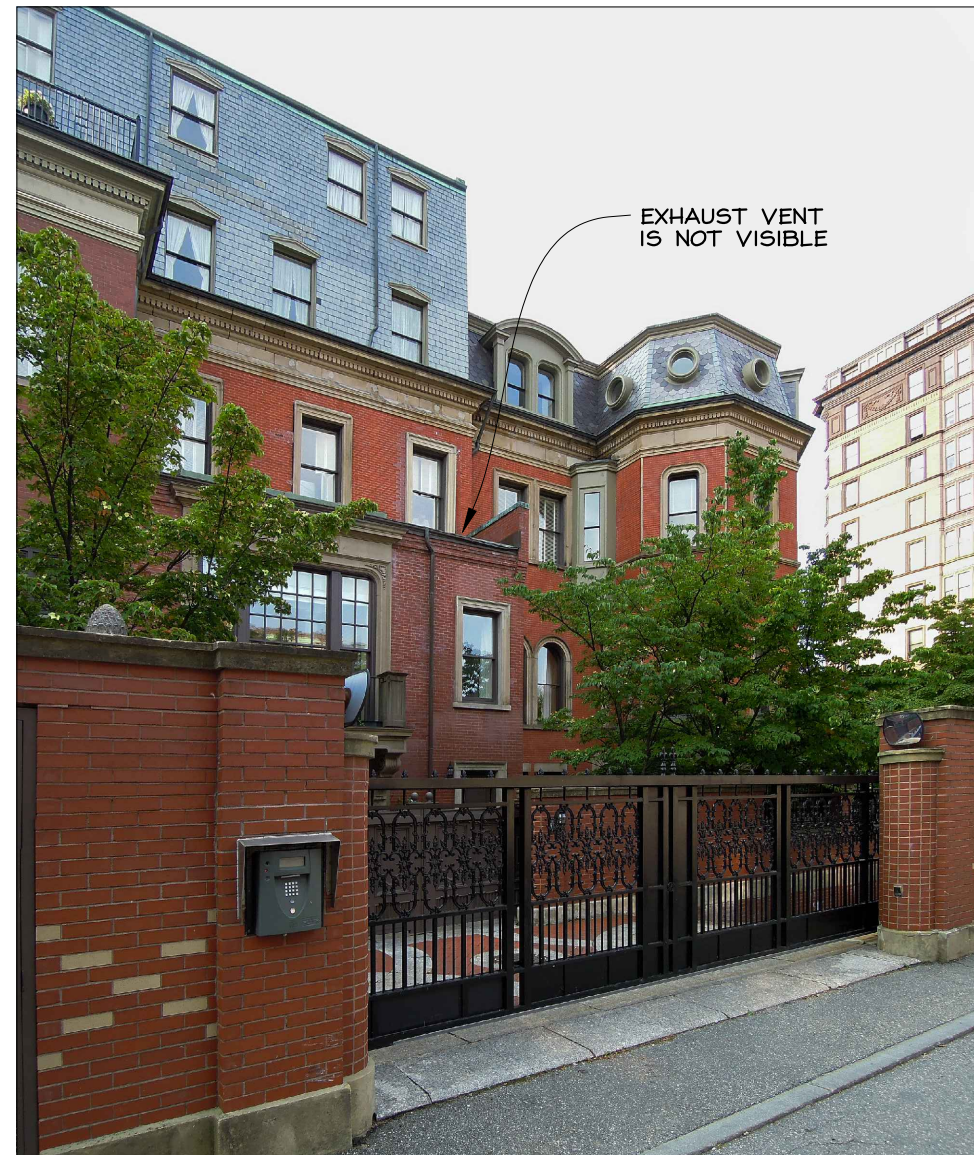
2 EXISTING CONDITIONS, VIEW FROM ALLEY LOOKING SOUTHWEST Not to Scale
