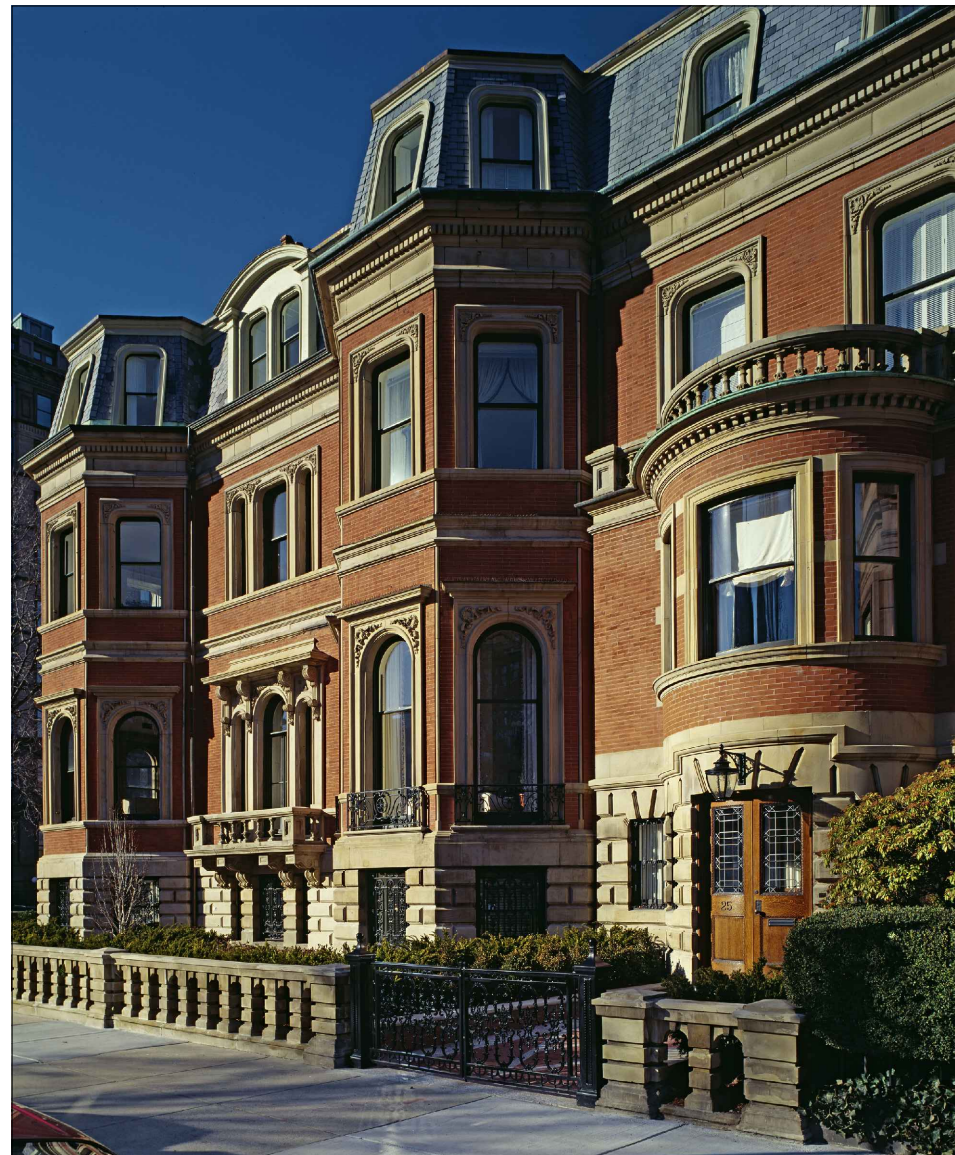
1 EXISTING CONDITIONS, VIEW OF FRONT ENTRY AT 25 COMMONWEALTH AVENUE Not to Scale
