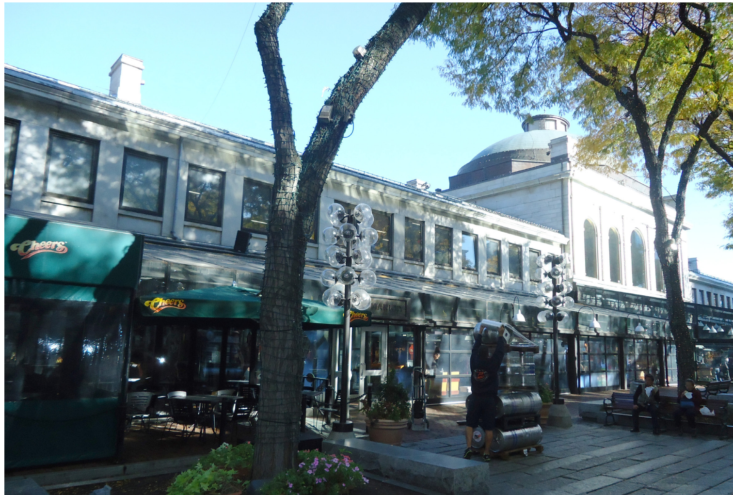
EXISTING EXTERIOR _ CLOSED CONDITION
