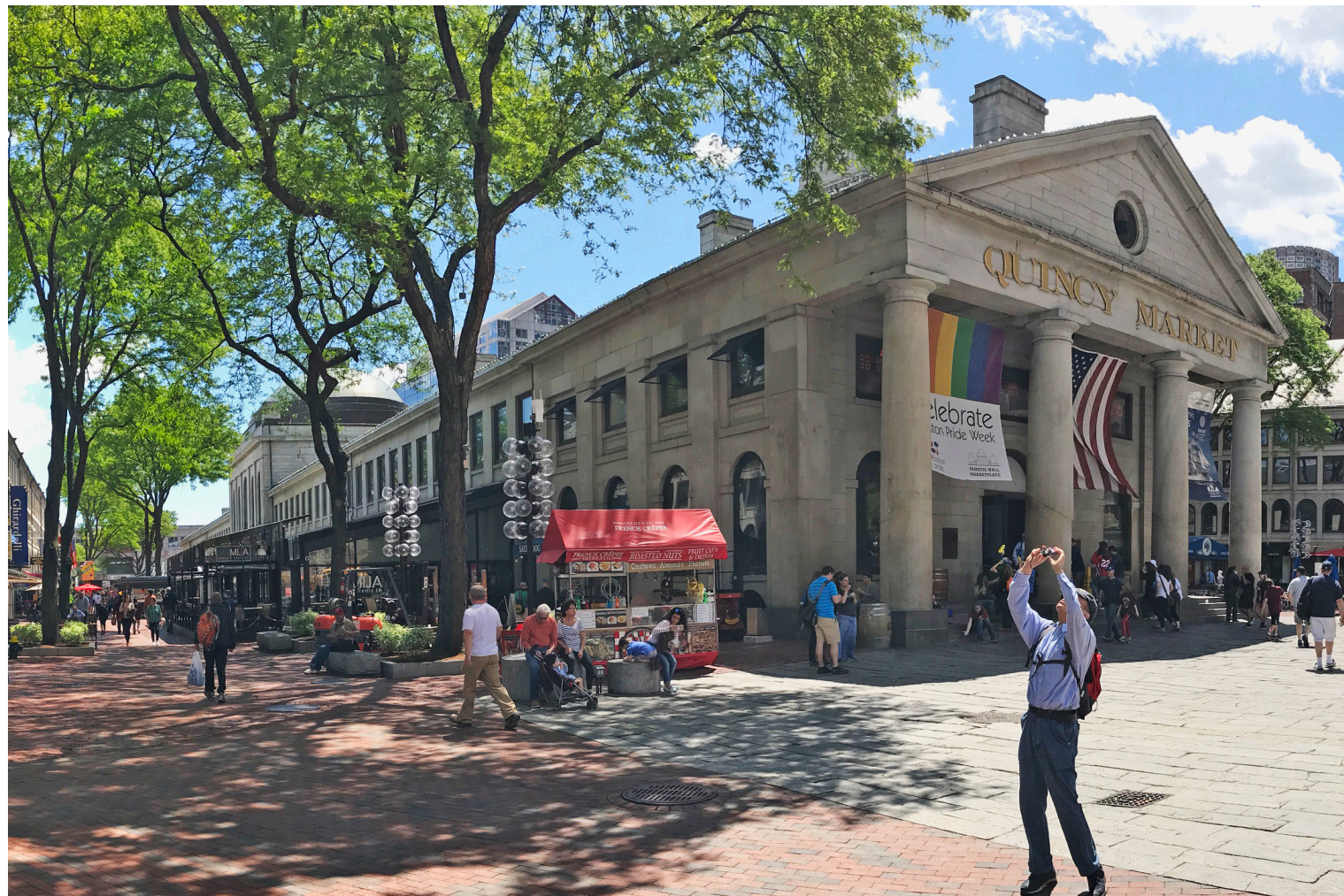
EXISTING - SITE PHOTO
