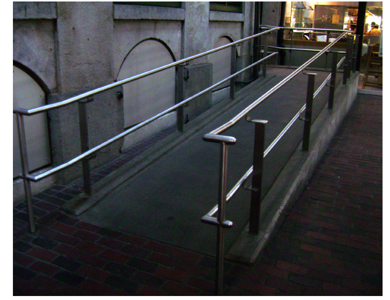
EXISTING QUINCY MARKET RAMP
