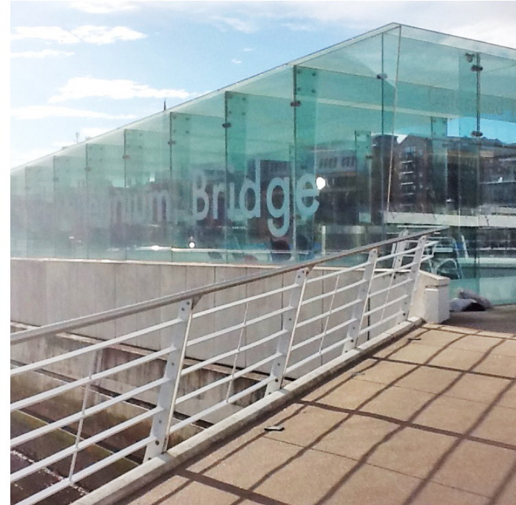
GATESHEAD MILLENNIUM BRIDGE, ENGLAND
