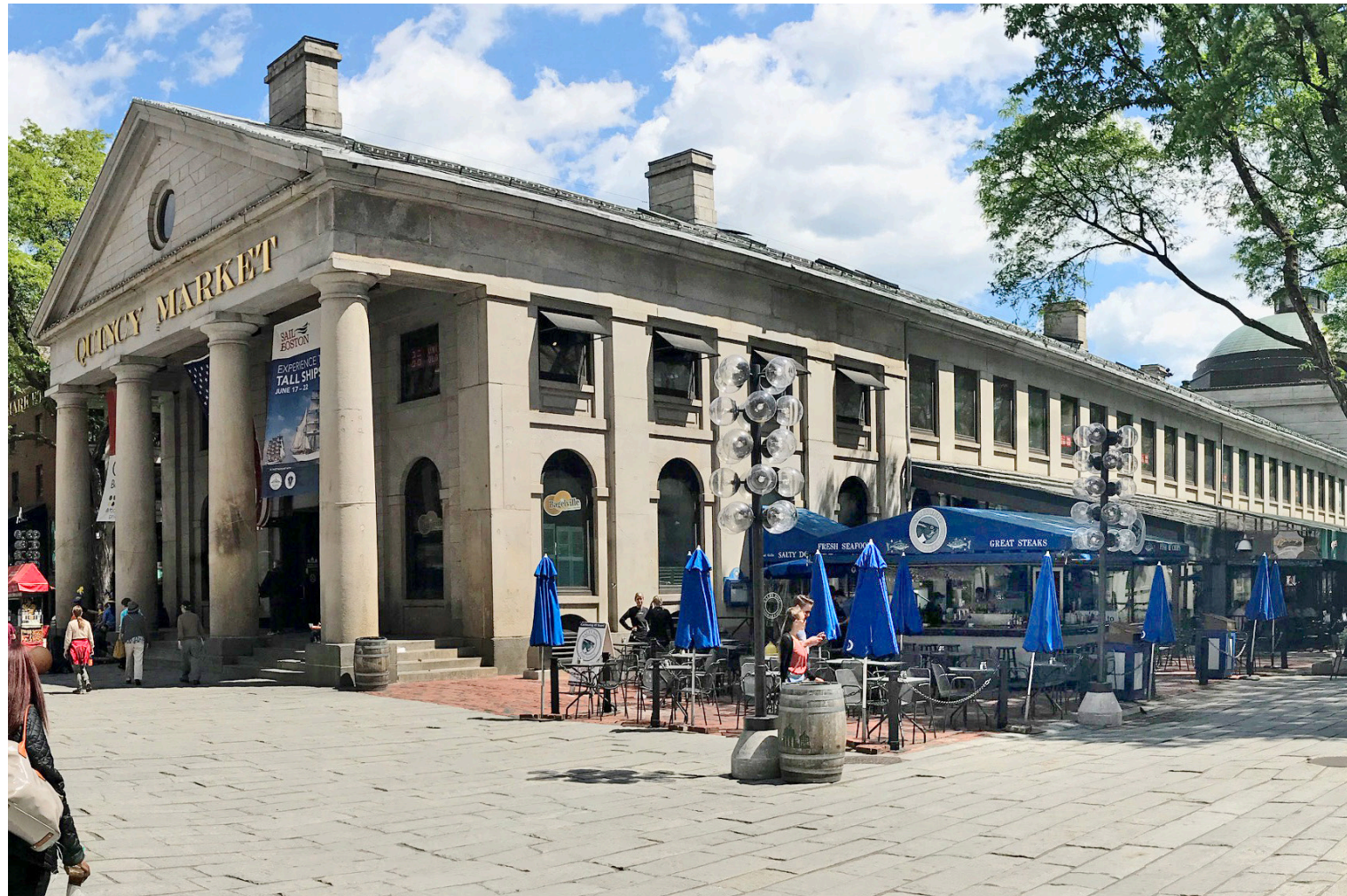
EXISTING - SITE PHOTO
