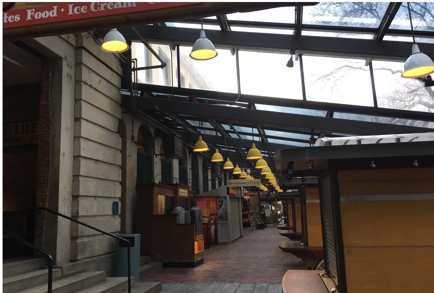
EXISTING CONDITION_ INTERIOR _LOOKING EAST
