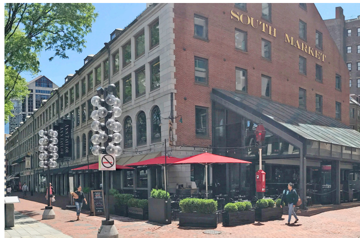
EXISTING - SITE PHOTO
