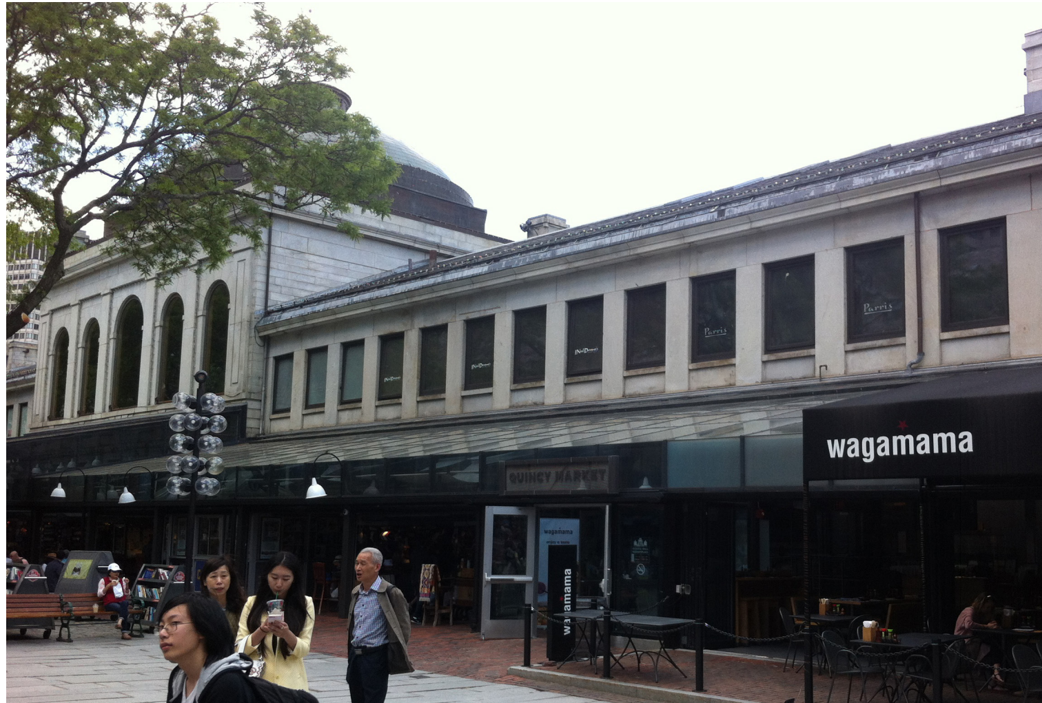
EXISTING CONDITION _ EXTERIOR _ LOOKING WEST
