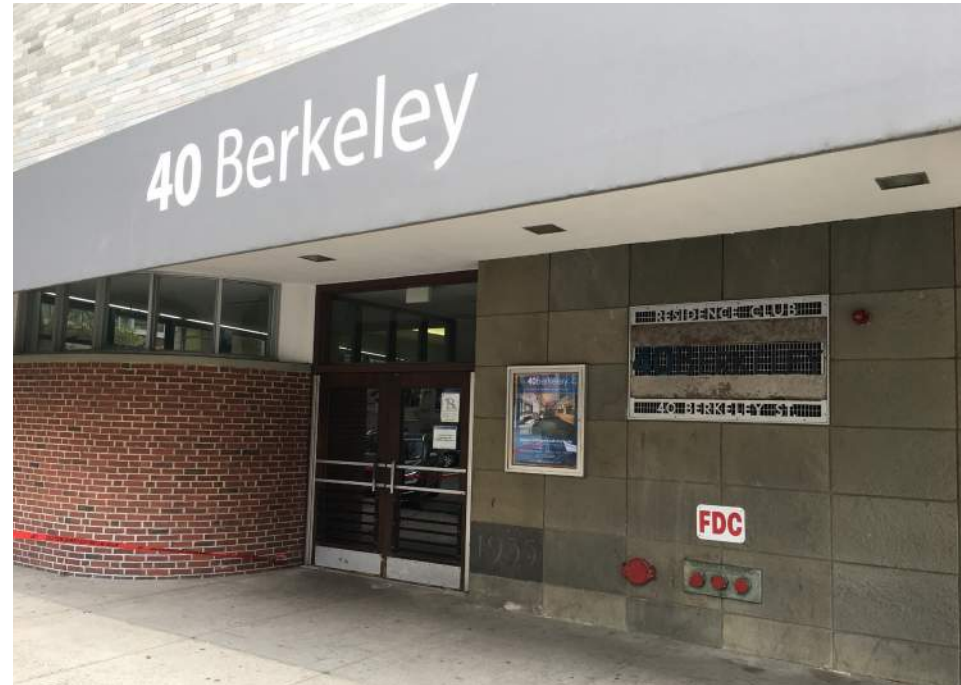
Berkeley Street Entry Canopy Lighting
