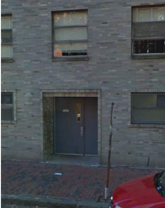
Appleton Street Access Door - Replace in kind
