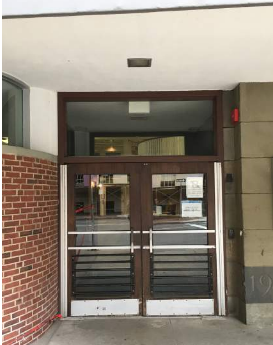
Berkeley Street Entrance Door - Refurbish
