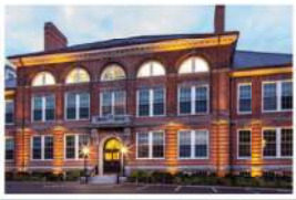
Kawneer: AA™5450 Series – OptiQ™ Ultra Thermal Windows Traco: NX-3800 fixed windows (curved) Coddington Hall, Quincy, Massachusetts Architect: Wessling Architects, Quincy, Massachusetts Window Installer: North East Energy Control Systems, Canton, Massachusetts Photography: © Bob Perzel
