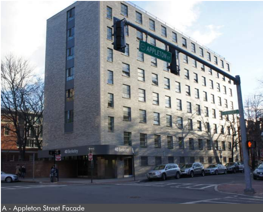
A - Appleton Street Facade
