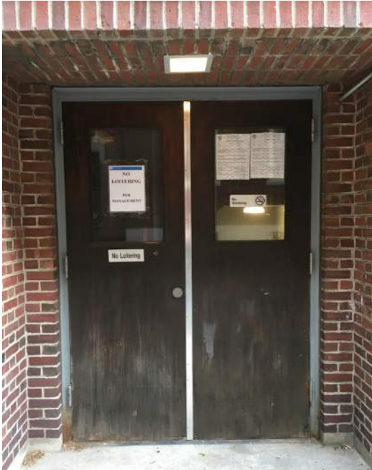
Grey Street Stair Door - Refurbish
