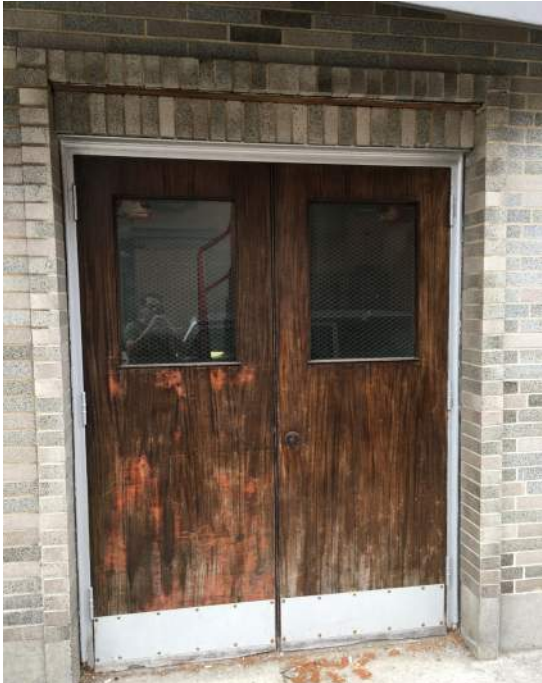
Appleton Street Stair Door - Refurbish
