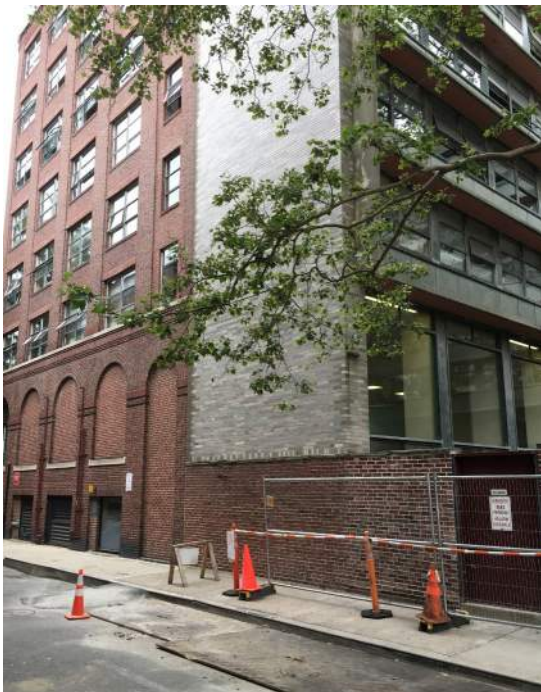
Grey Street Facade
