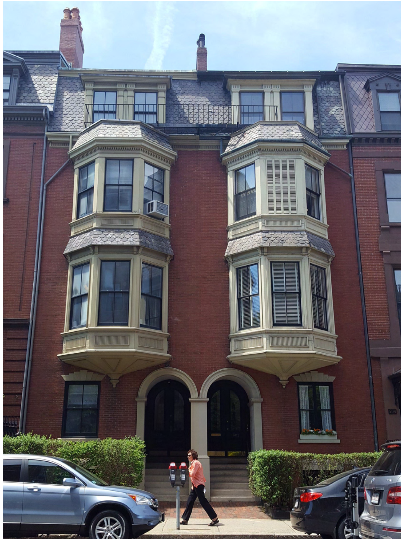
FRENCH CULTURAL CENTER 53 MARLBOROUGH / 300 BERKELEY STREET
