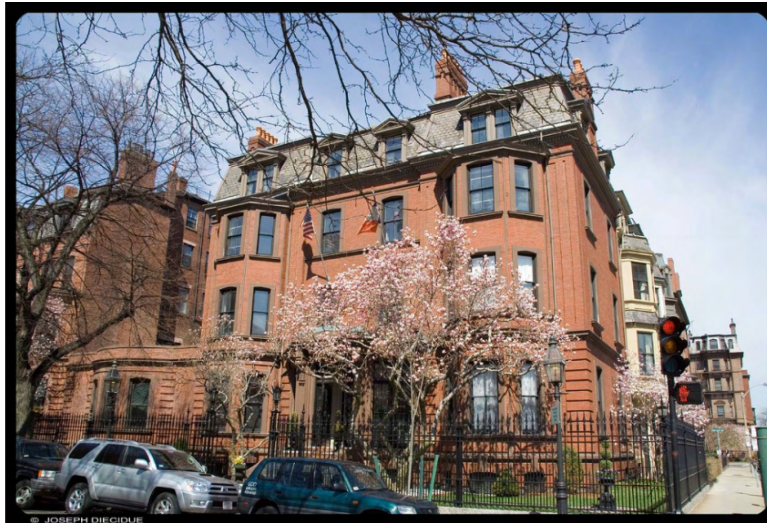
FRENCH CULTURAL CENTER 53 MARLBOROUGH / 300 BERKELEY STREET 6.20.2017
