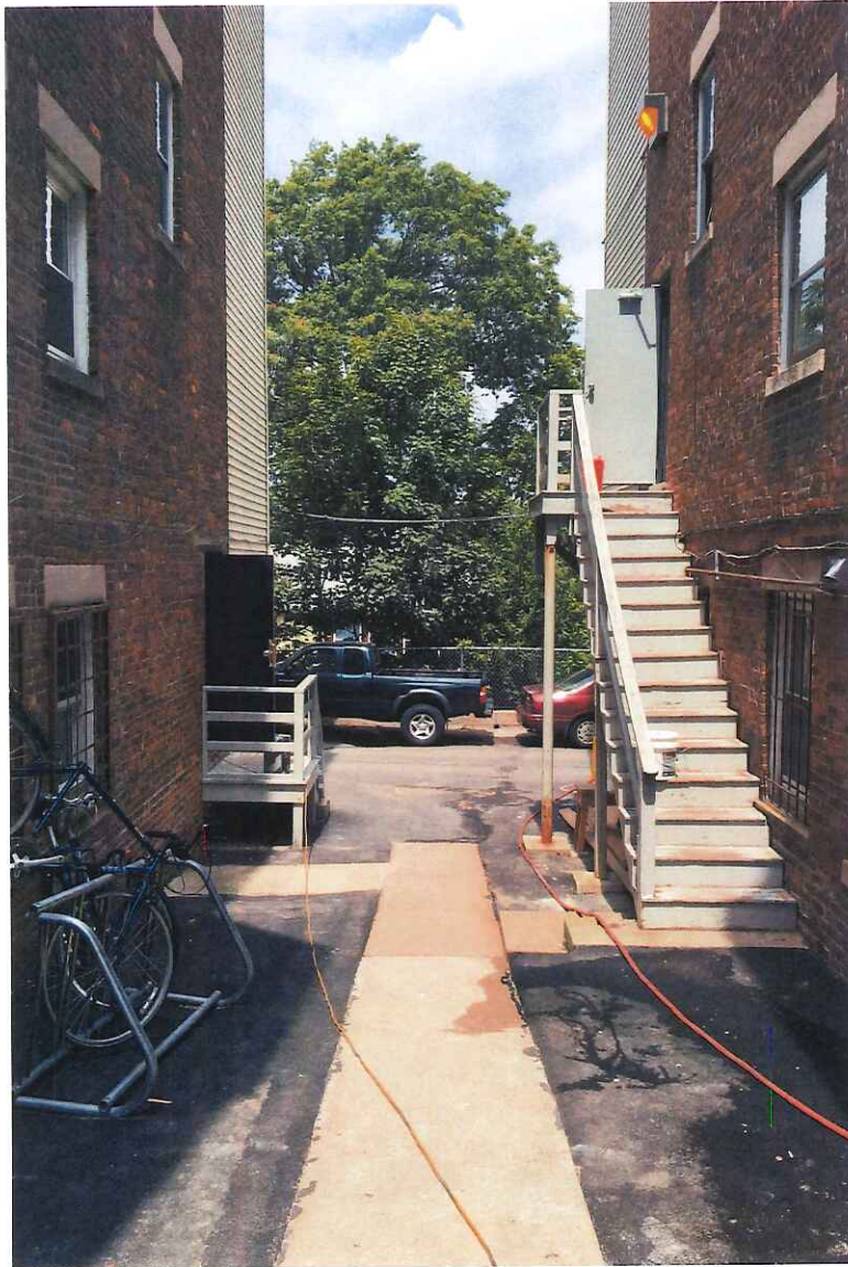
EXISTING STAIR 'B' & 'C'
