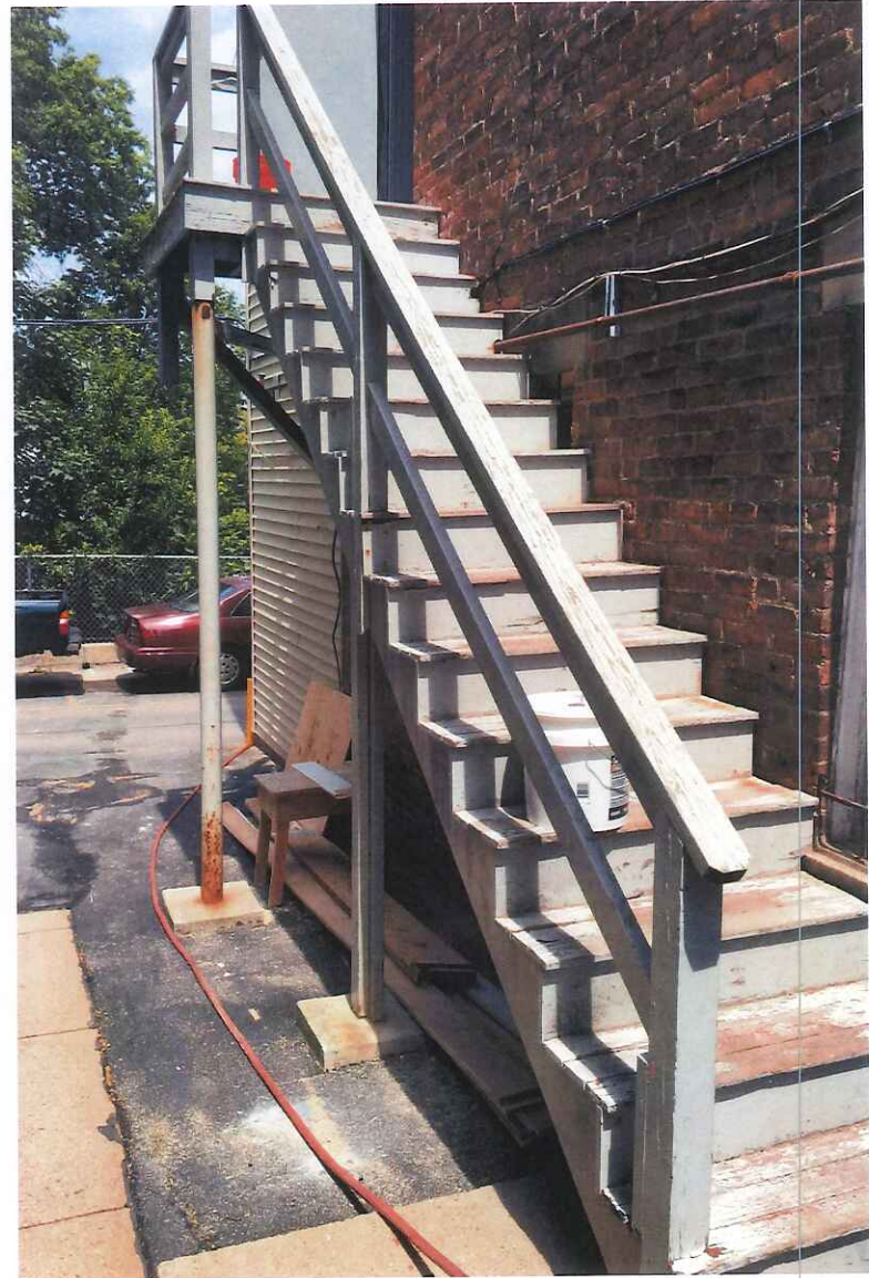
EXISTING STAIR 'C'
