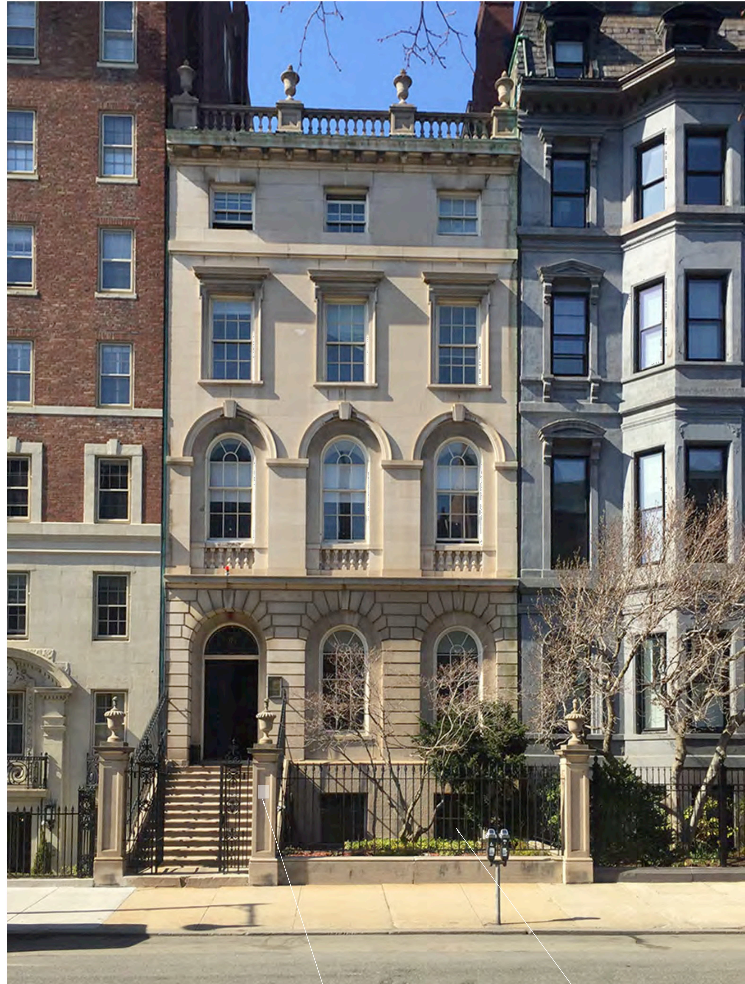
1 PHOTO - EXISTING FRONT FACADE AND FRONT YARD @ 170 BEACON STREET SCALE: N/A
