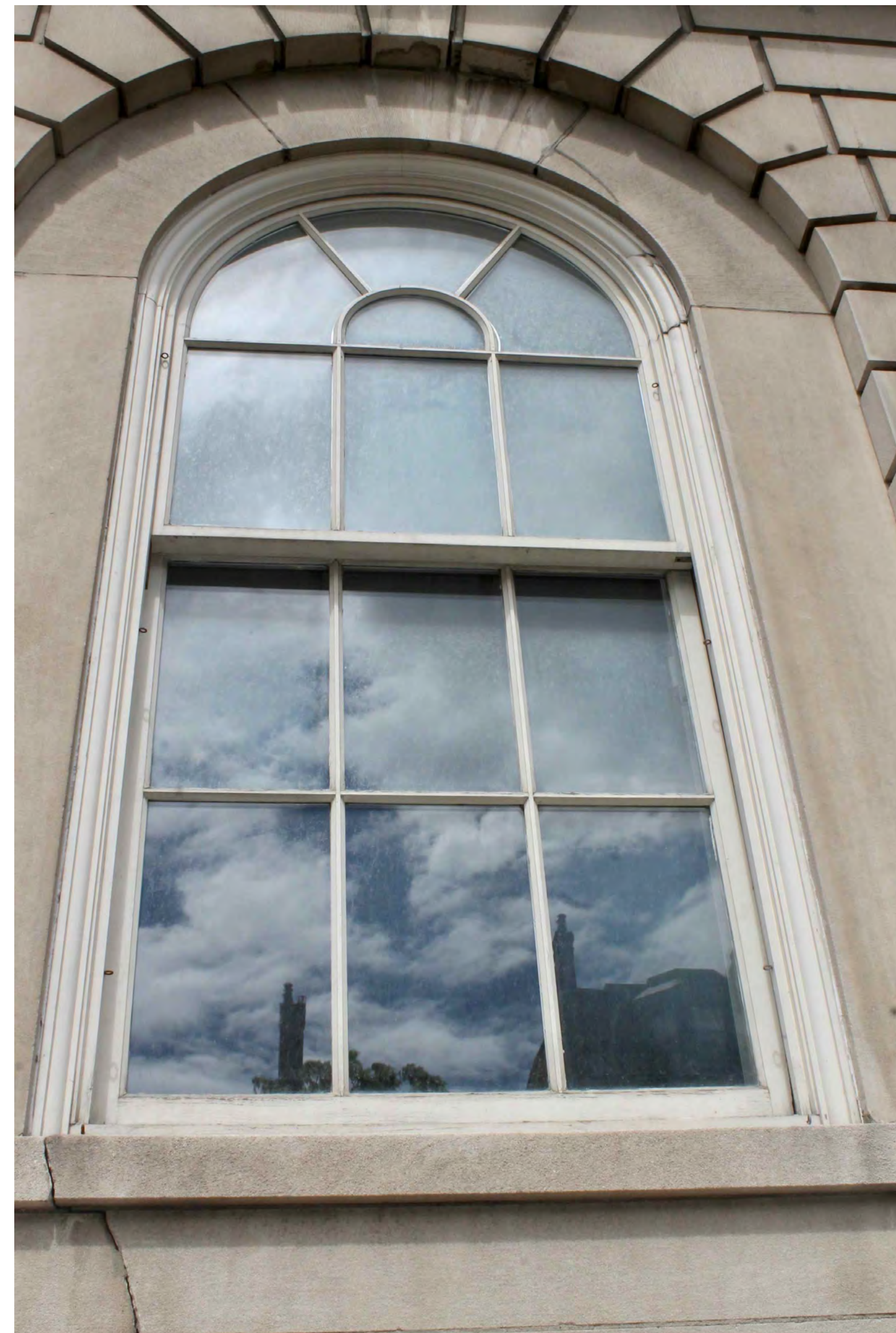
WOOD WINDOW (c. 1989) TO BE REPLACED IN-KIND
