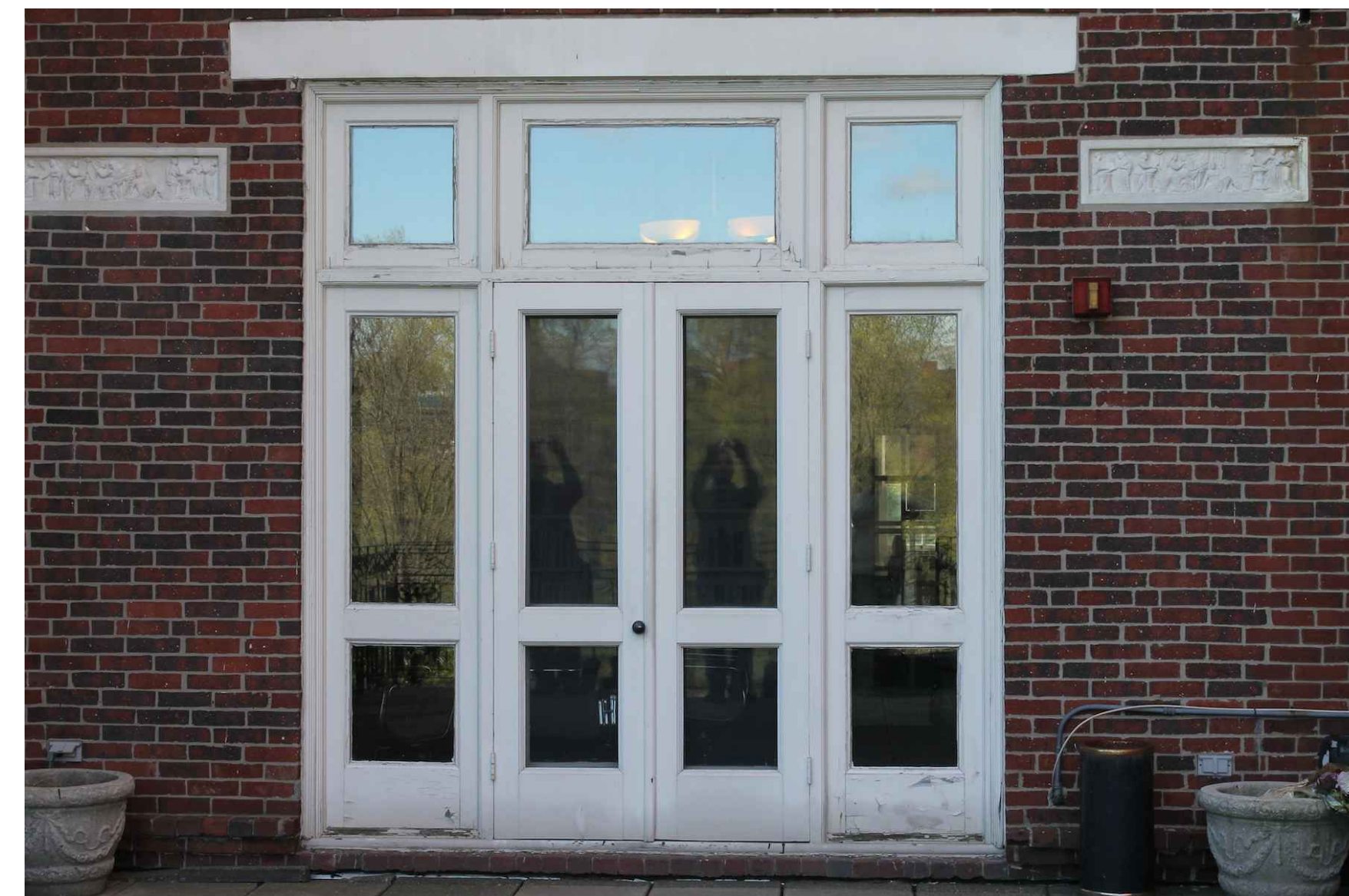
2ND FLOOR DOOR UNIT TO TERRACE – REPAIR ONLY
