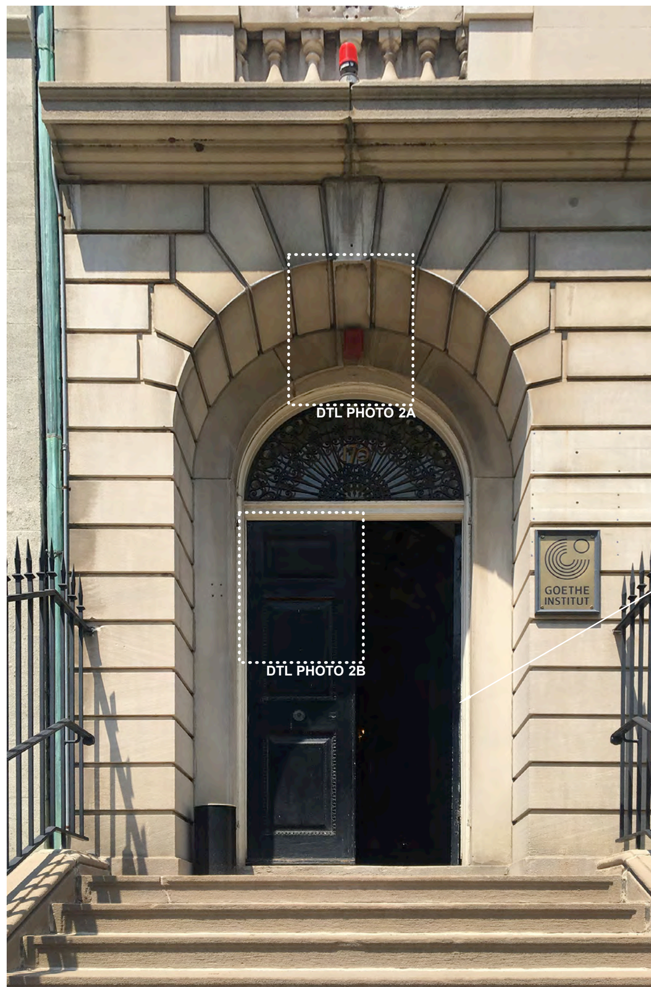
3 PHOTO - EXISTING PUBLIC FRONT ENTRANCE SCALE: N/A
