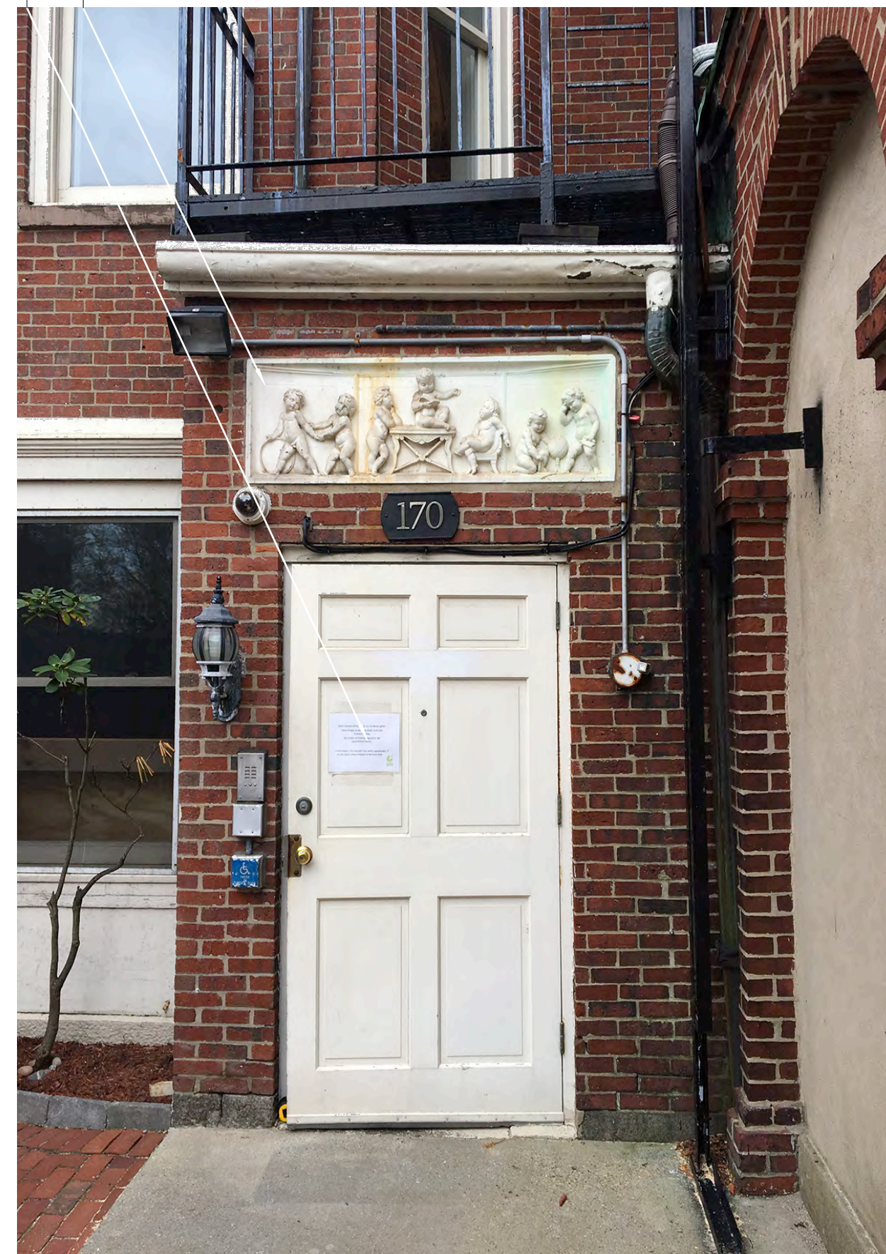
2 PHOTO - EXISTING ACCESSIBLE PUBLIC ENTRANCE SCALE: N/A
