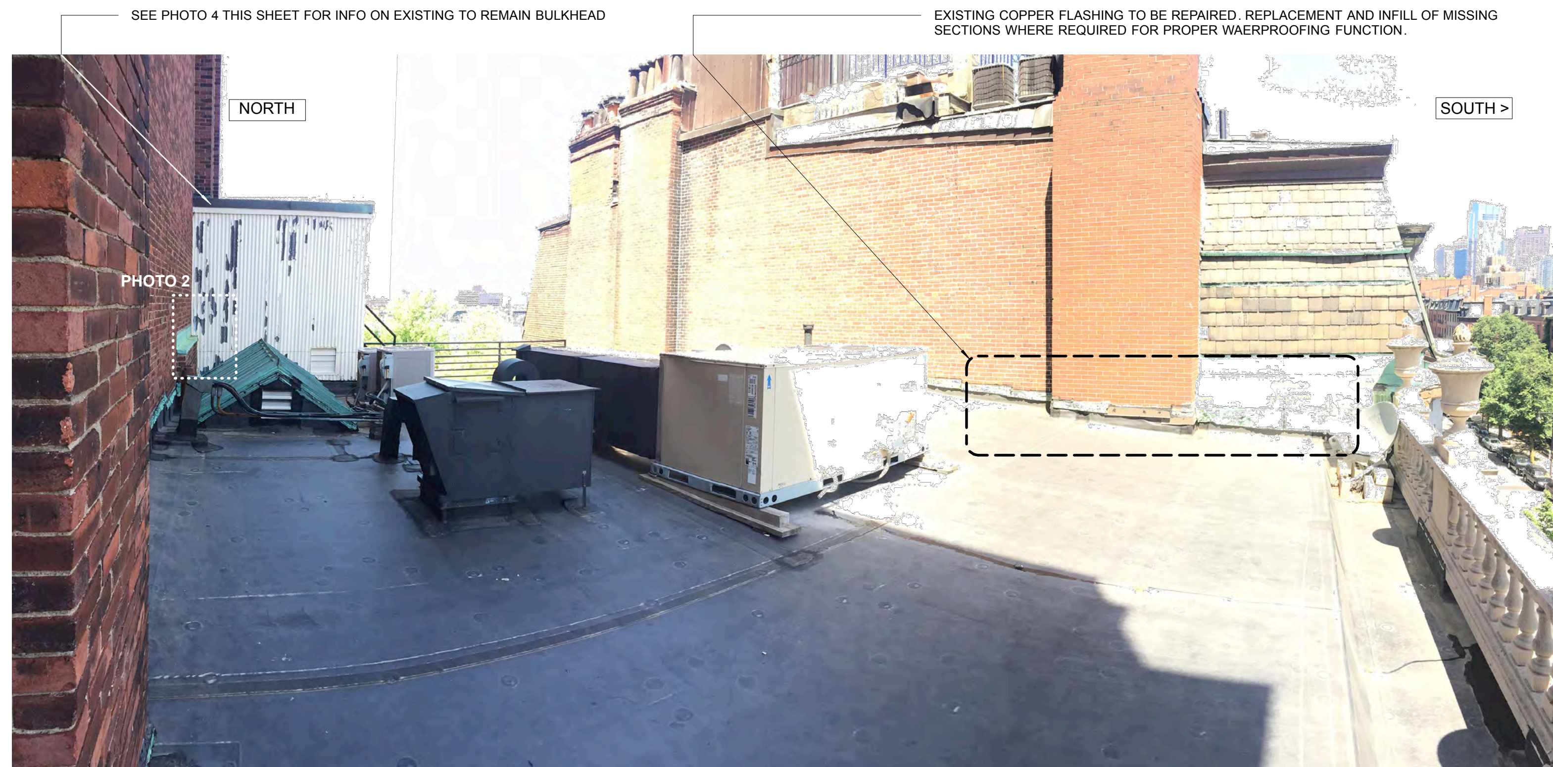
1 PHOTO - EXISTING HIGH ROOF, ELEVATOR MACHINE ROOM BULKHEAD + MECHANICAL EQUIPMENT SCALE: N/A
