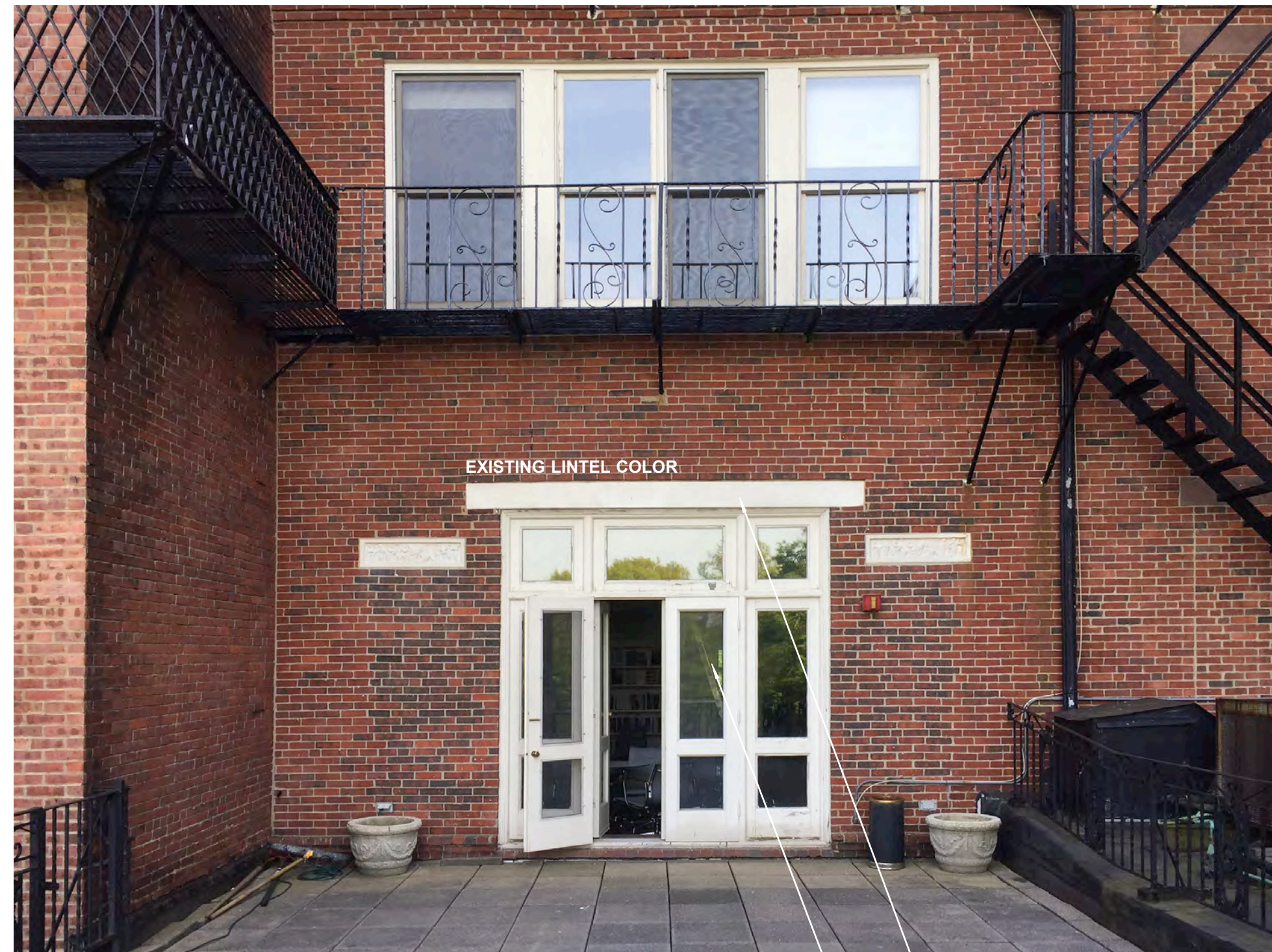
5 PHOTO - EXISTING 2ND FLOOR TERRACE SCALE: N/A
