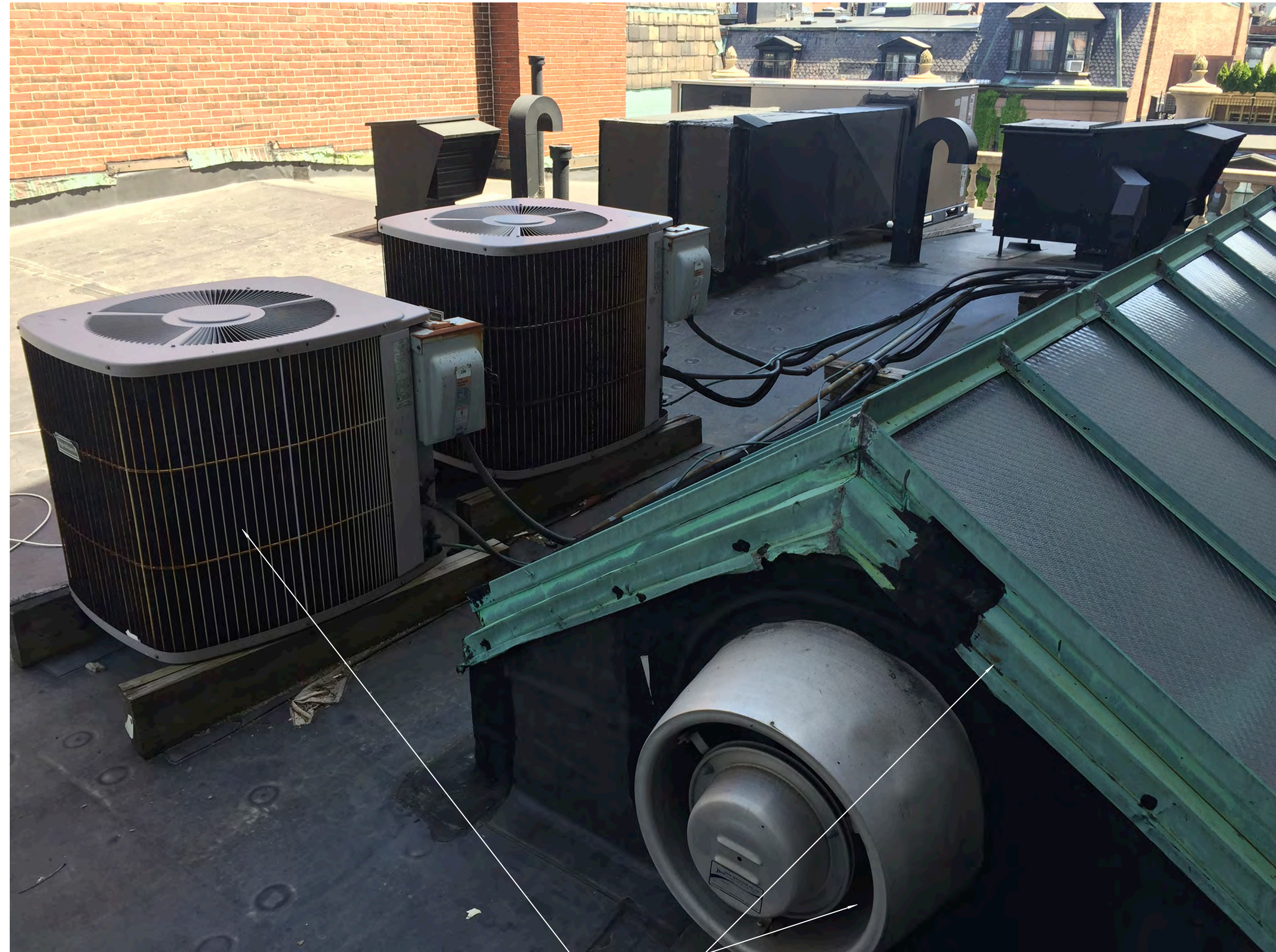
3 PHOTO - EXISTING MECHANICAL EQUIPMENT + SKYLIGHT SCALE: N/A
