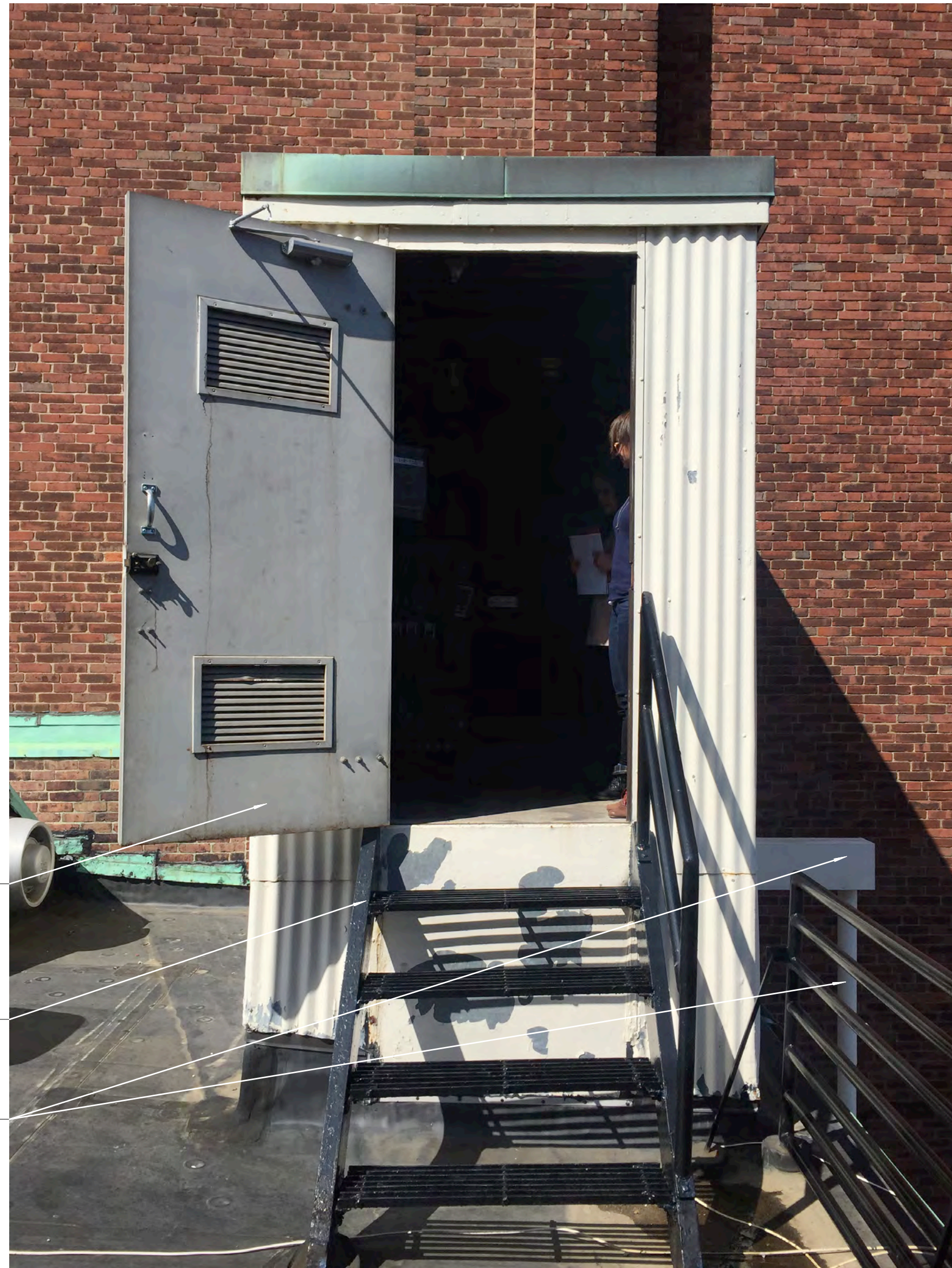
4 PHOTO - EXISTING ELEVATOR MACHINE ROOM BULKHEAD SCALE: N/A
