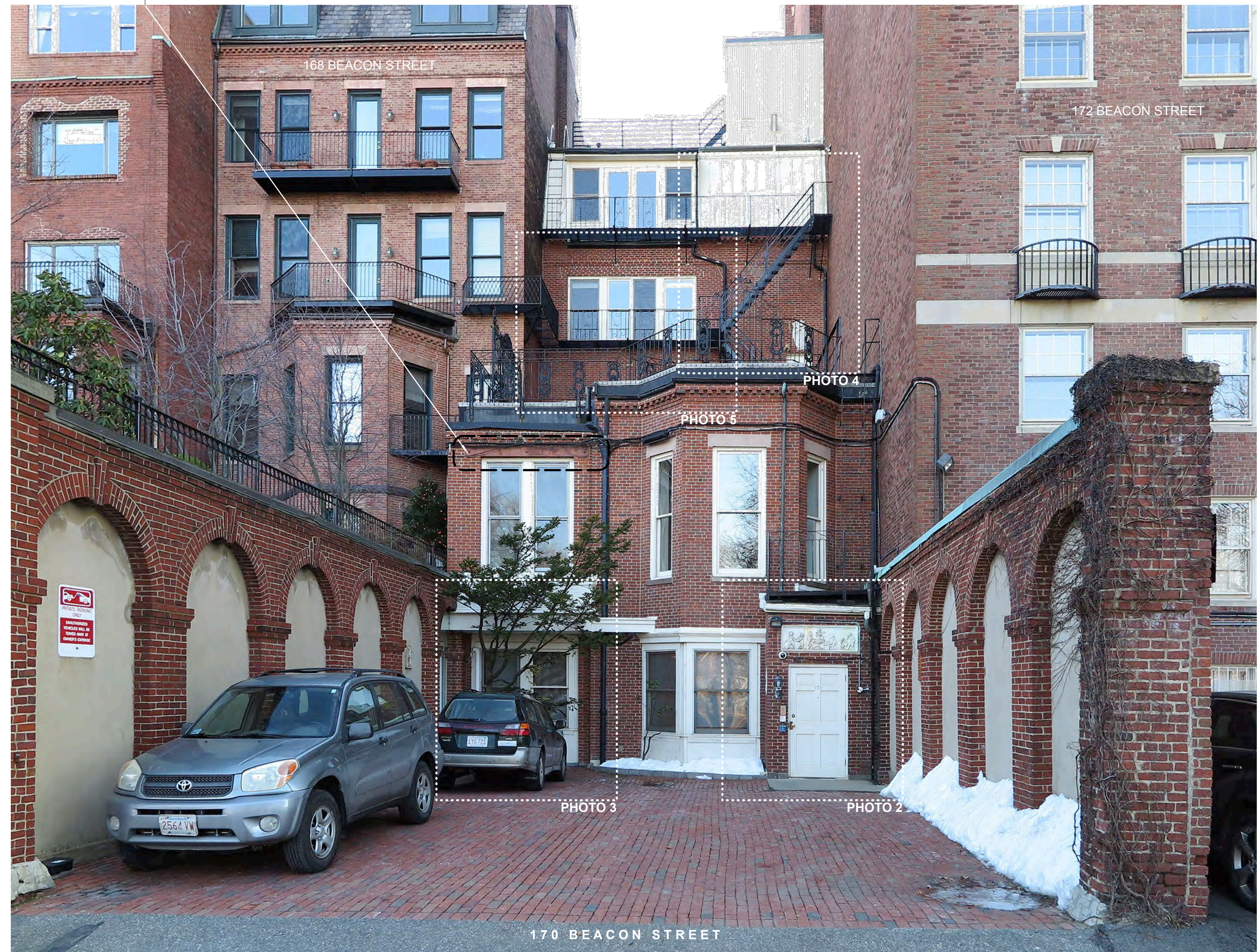
1 PHOTO - EXISTING REAR FACADE AND REAR YARD SCALE: N/A
