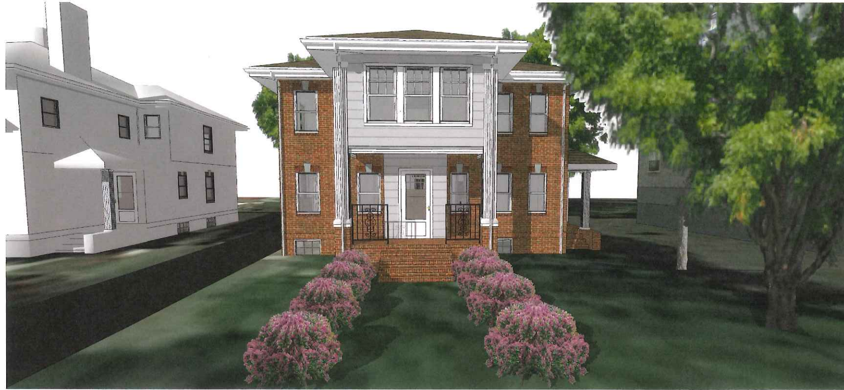
Front Facade, Existing
