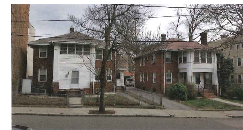
3 Front Facade, Spring 101-103 Kilsyth on right
