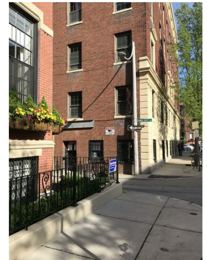
PUBLIC ALLEY 415 FACADE AT GLOUCESTER ST
