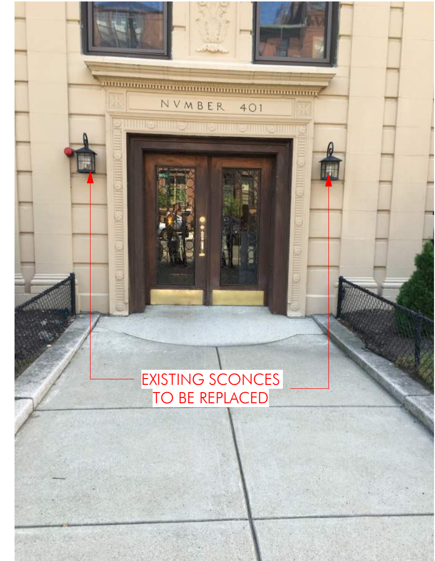
BEACON STREET FACADE - EXISTING SCONCES
