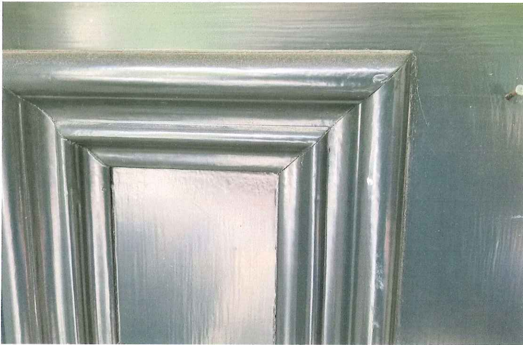
Close Up of Door Molding (for reference)
