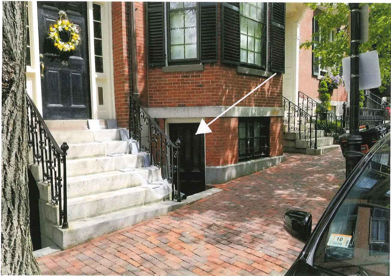
Location of Door to be Modified - Lower Level - 43 Chestnut Street
