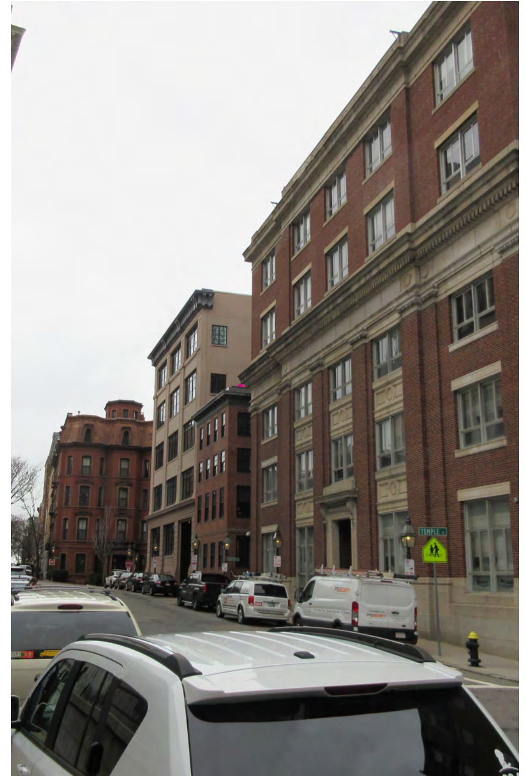
3 From Derne St at Garage Entry
