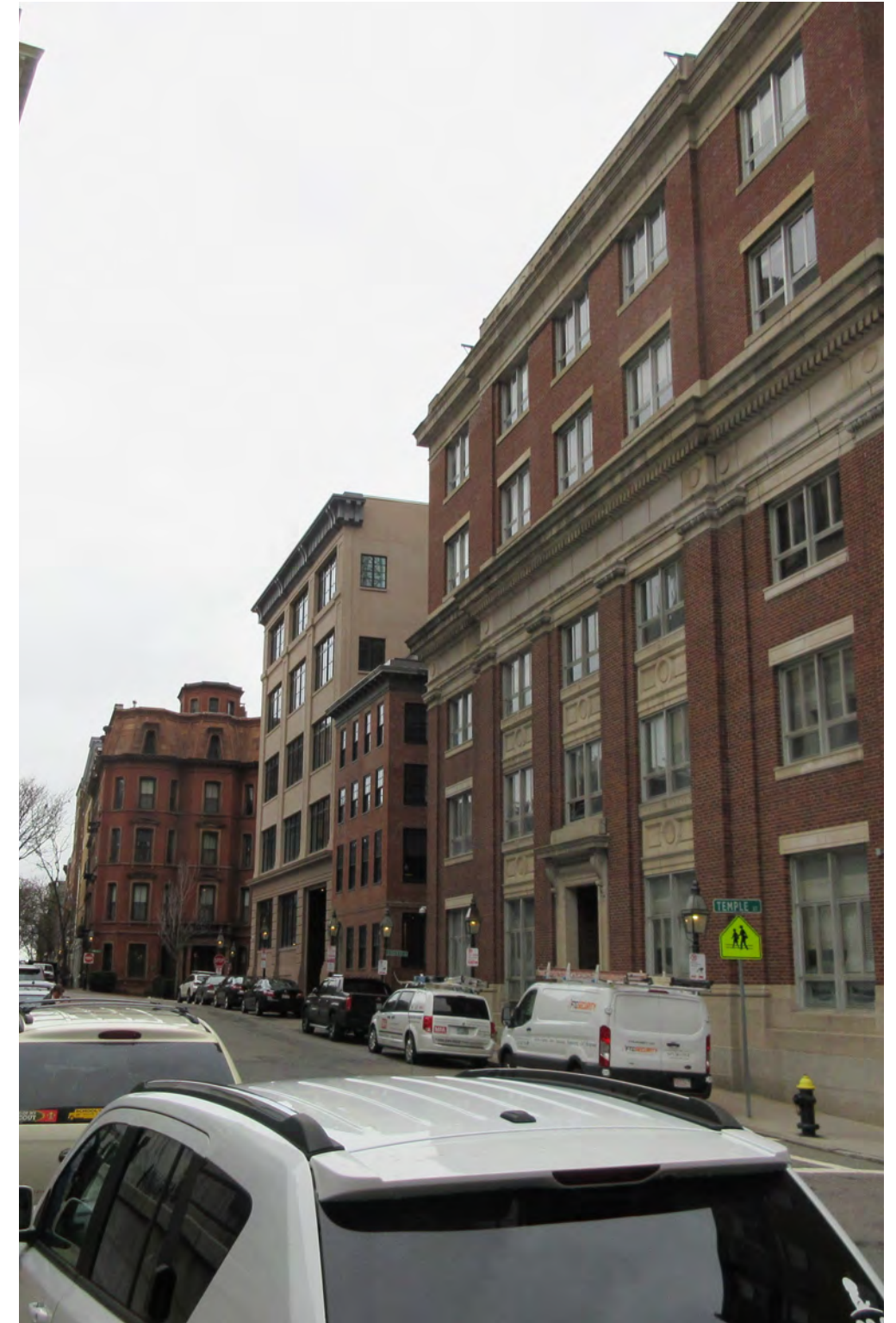
3 From Derne St at Garage Entry
