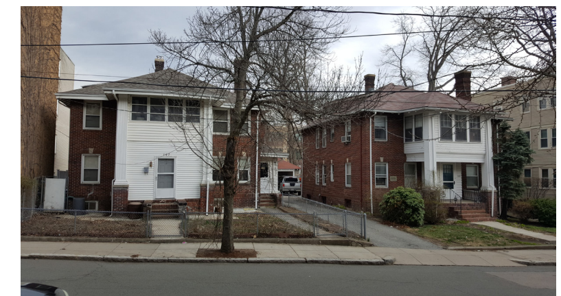
3 Front Facade, Spring 101-103 Kilsyth on right
