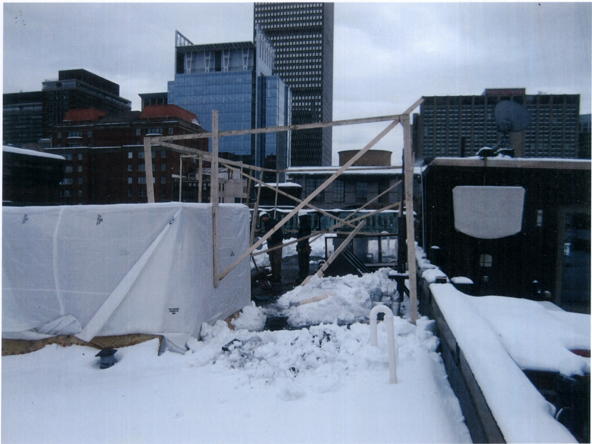
284 COMM. AVE. - MEZZANINE MOCK UP (LOOKING SE)
