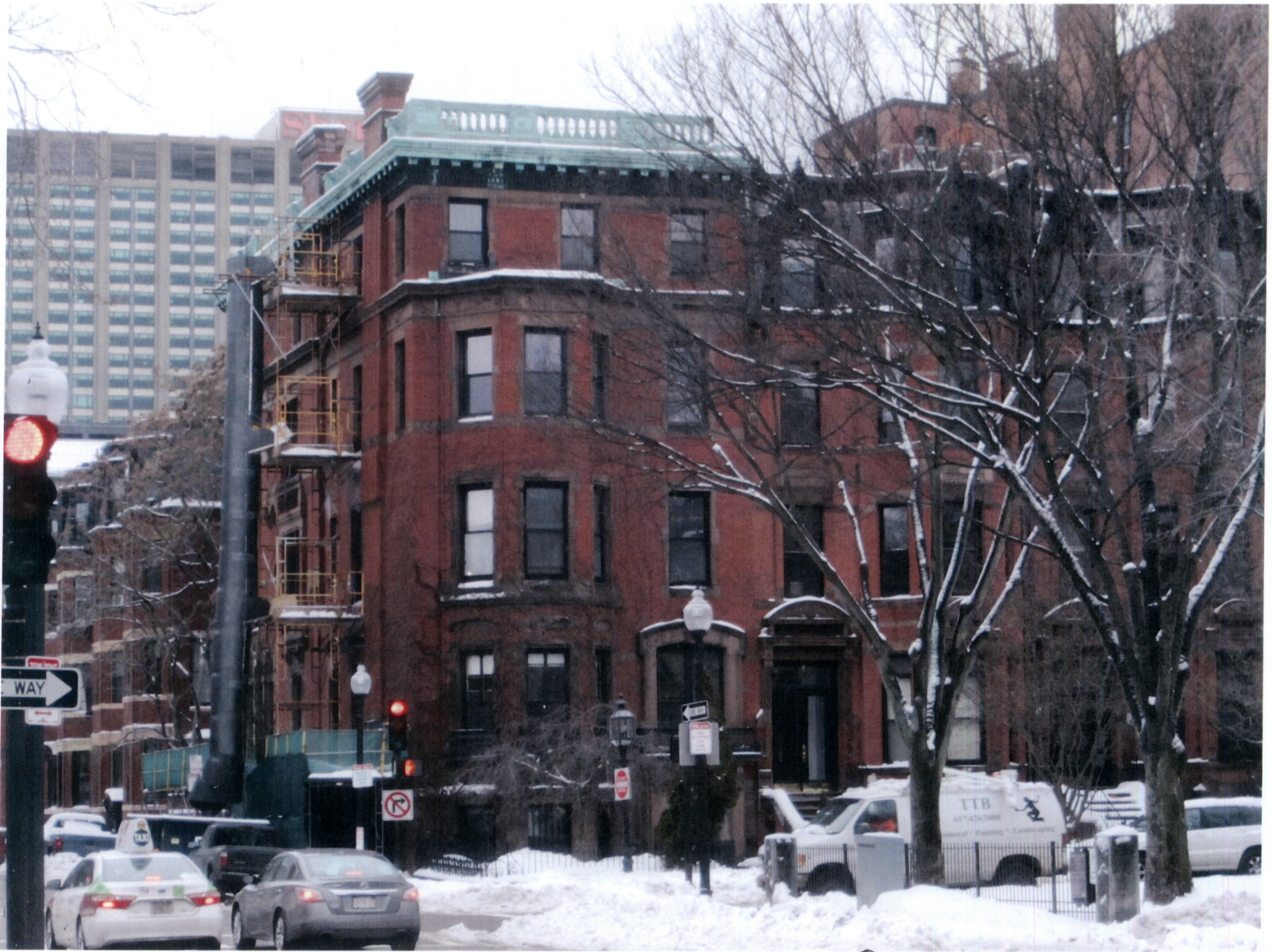
284 COMM. AVE. - PHOTO (C) MEZZANINE MOCKUP 02.13.17
