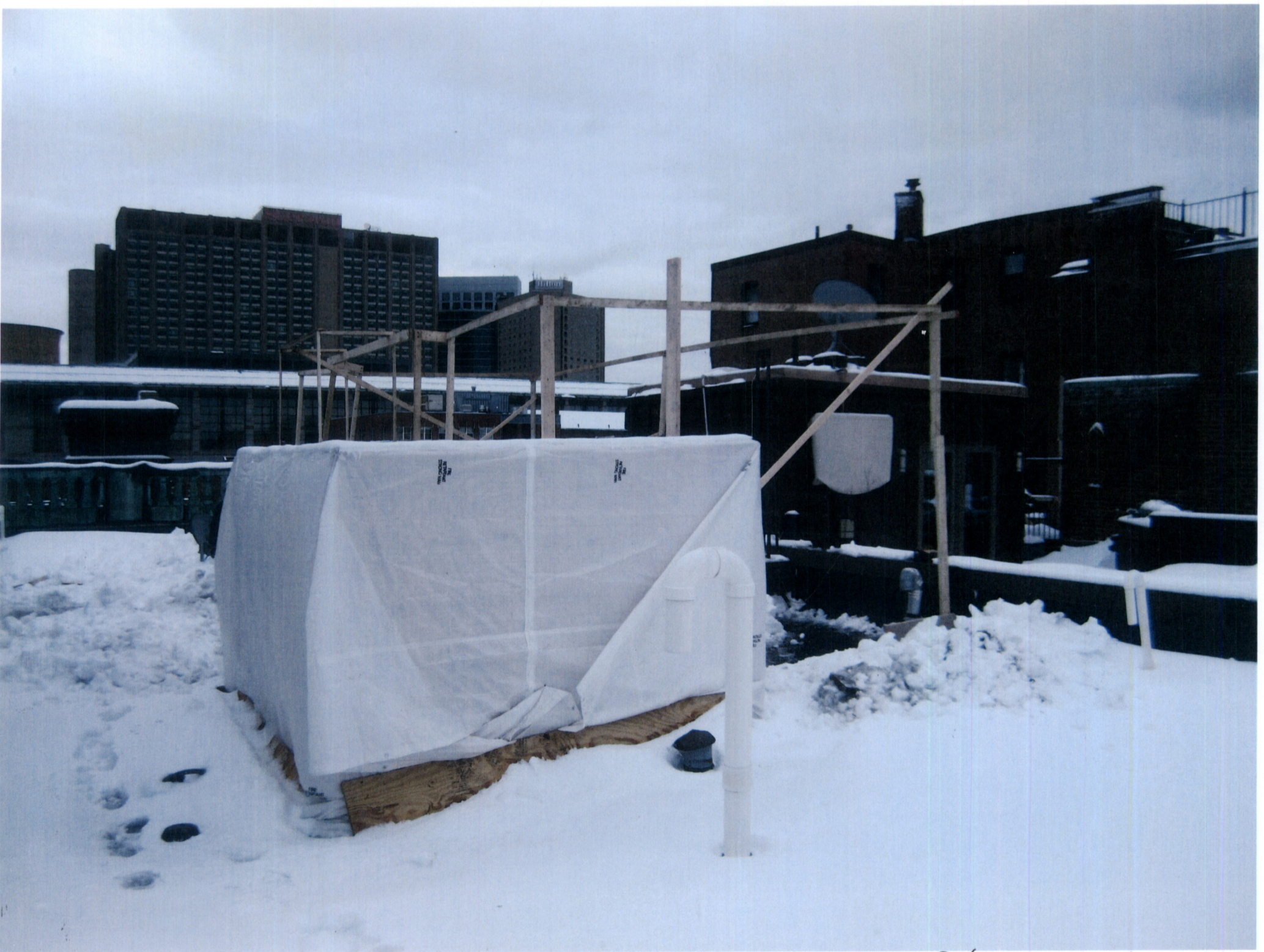
284 COMM. AVE. - MEZZANINE MOCK UP (LOOKING SOUTH) 02.13.17
