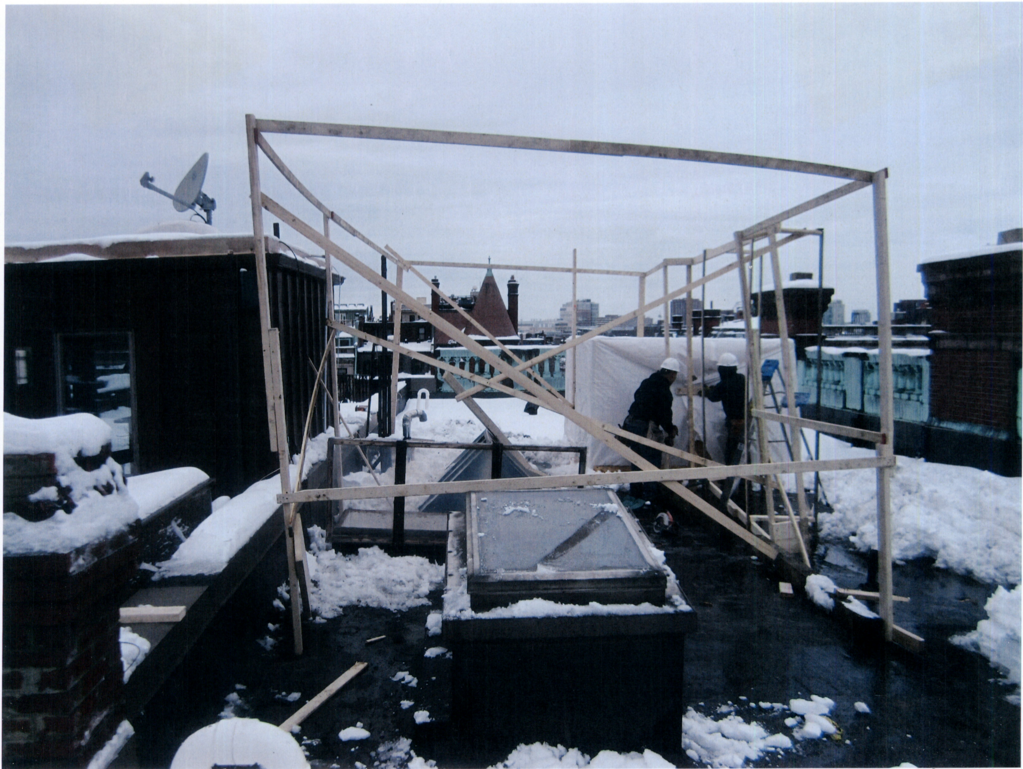
284 COMM. AVE. - MEZZANINE MOCK UP (LOOKING NORTH) 02.13.17
