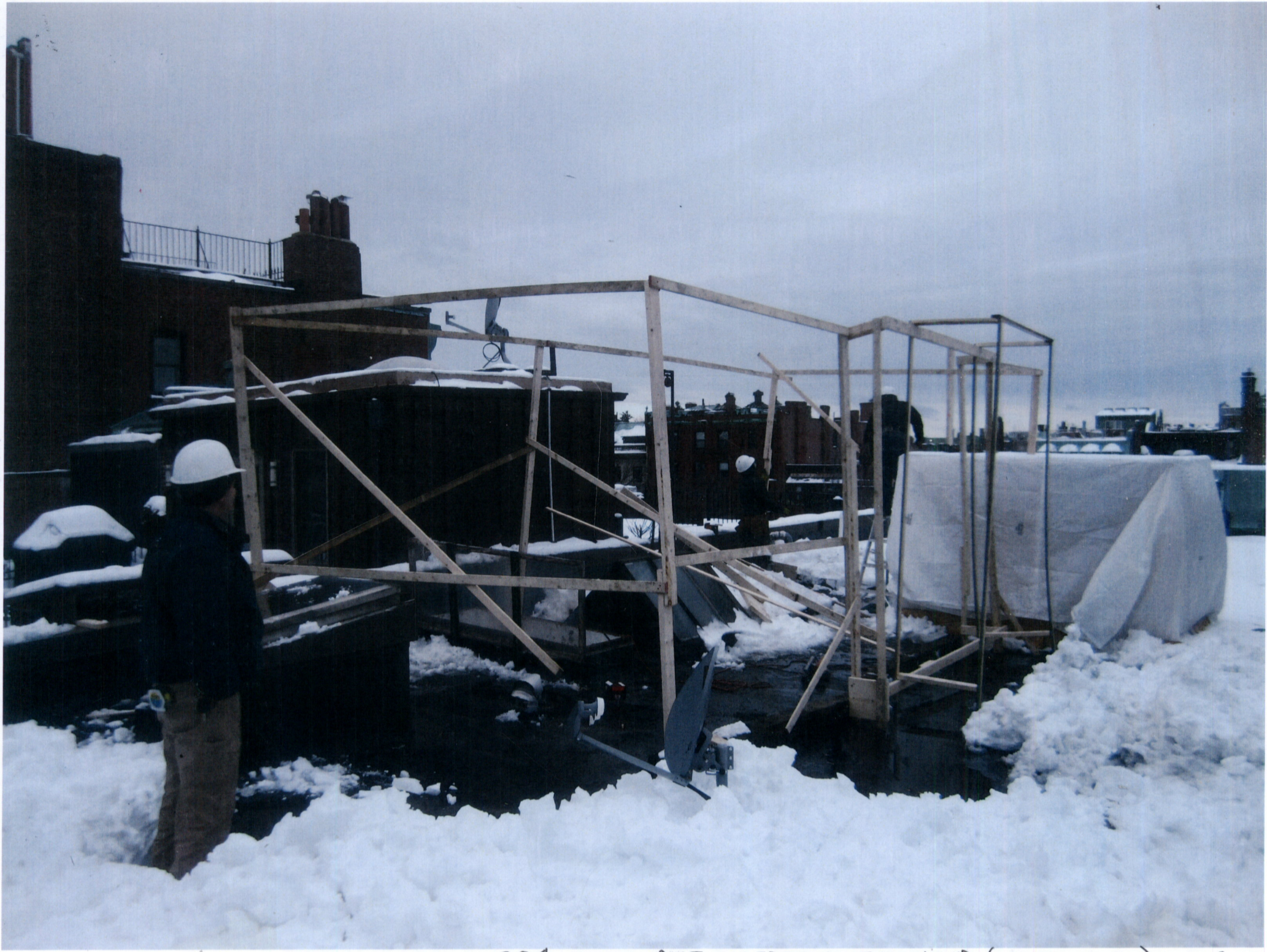
284 COMM. AVE. - MEZZANINE MOCK UP (LOOKING NW) 02.13.17
