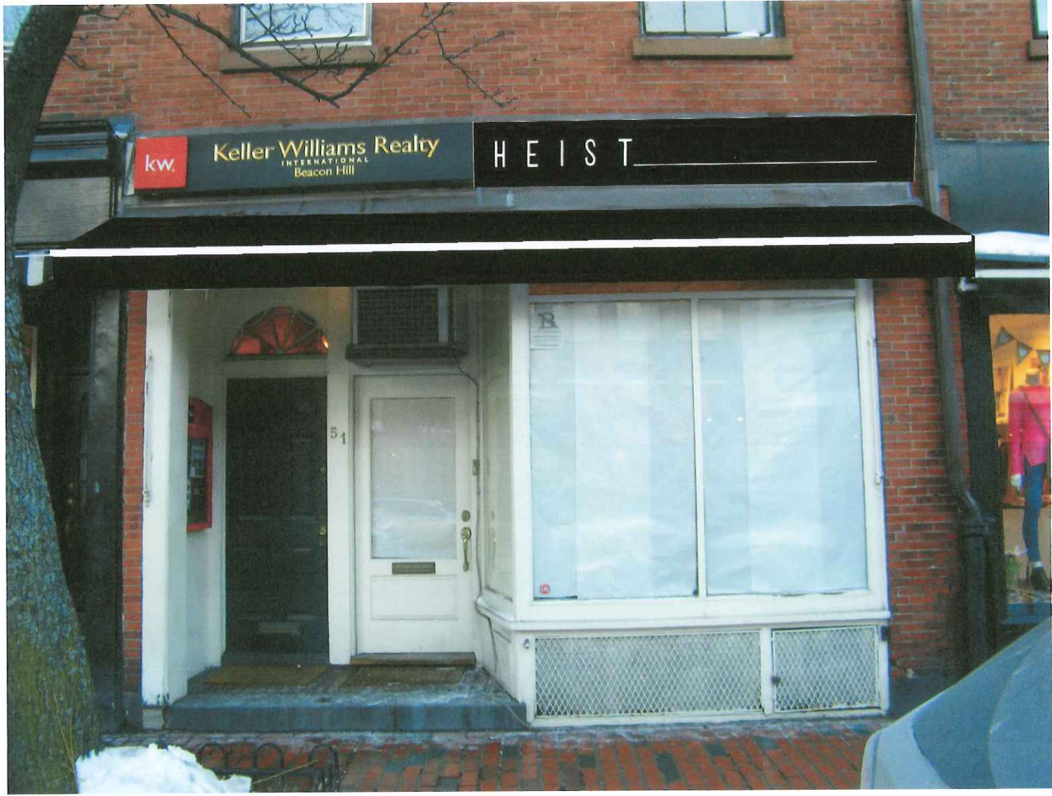
(A) Retractable Awning- Propose to recover existing roll out awning with new Sunbrella Black fabric for awning and valance. (9"). Awning measures 17' wide/ 5' projection. Wall Sign - One (1) 16" high by 9'-0" long by 1" deep matte black aluminum sign sign background with 1" deep raised white letters and underline reading "HEIST".
