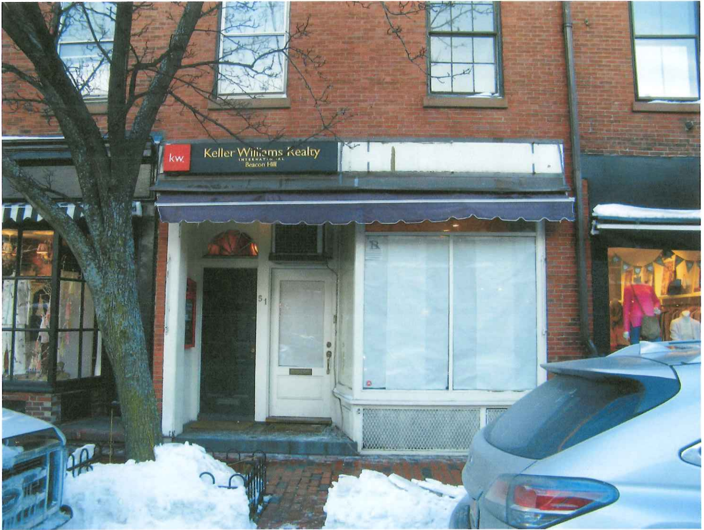
Photo of existing storefront, awning and sign area.
