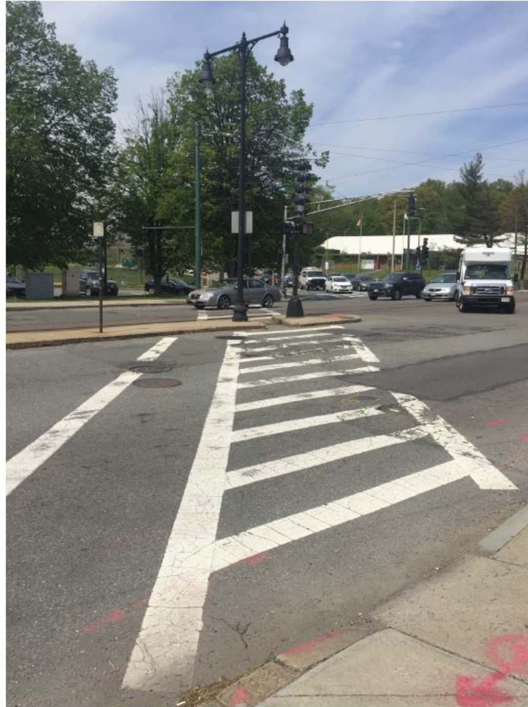
Figure 2 - Double Lamp to be Retained or Reset (Typ), Signal Post and Head to be Replaced (Typ), Mast Arm and Signal Heads to be Replaced (Typ)
