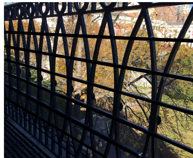
PROPOSED BALCONY METAL ROD MOCK-UP
