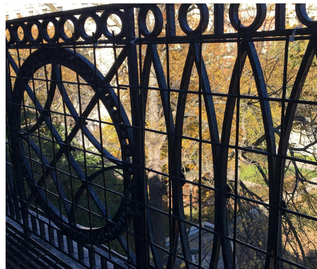
PROPOSED BALCONY WIRE MESH MOCK-UP
