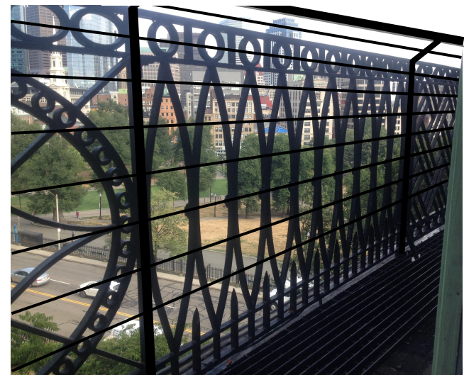
PROPOSED BALCONY POST & CABLE MOCK-UP
