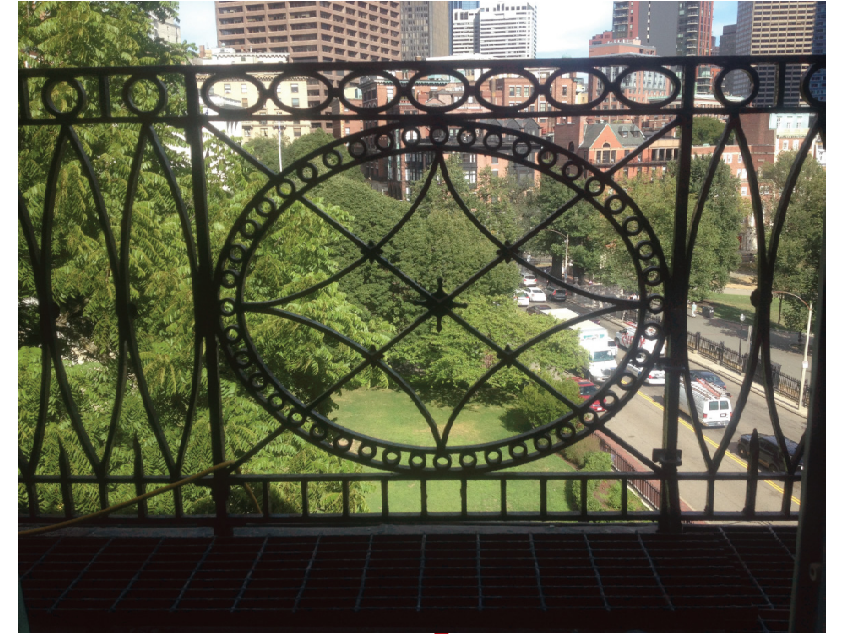
PARTIAL EAST RAILING
