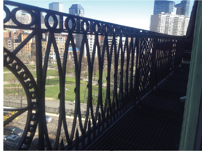
PARTIAL EAST RAILING
