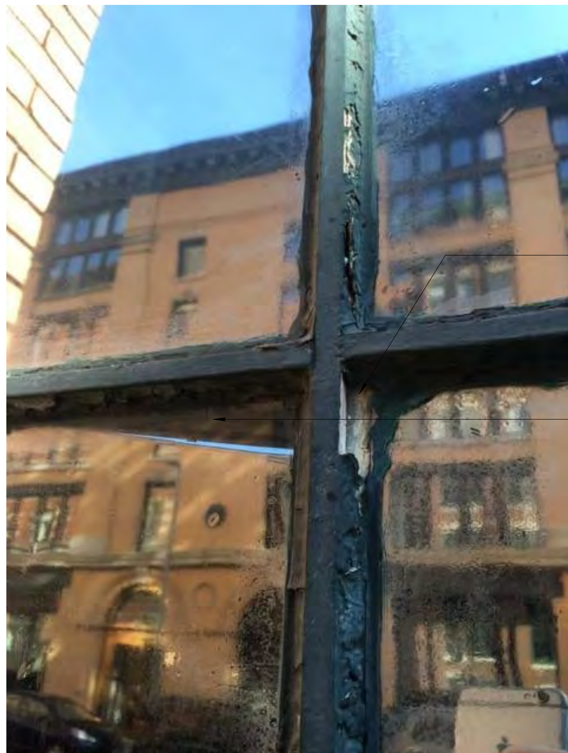
DAMAGED + ROTTING WOOD SILL
