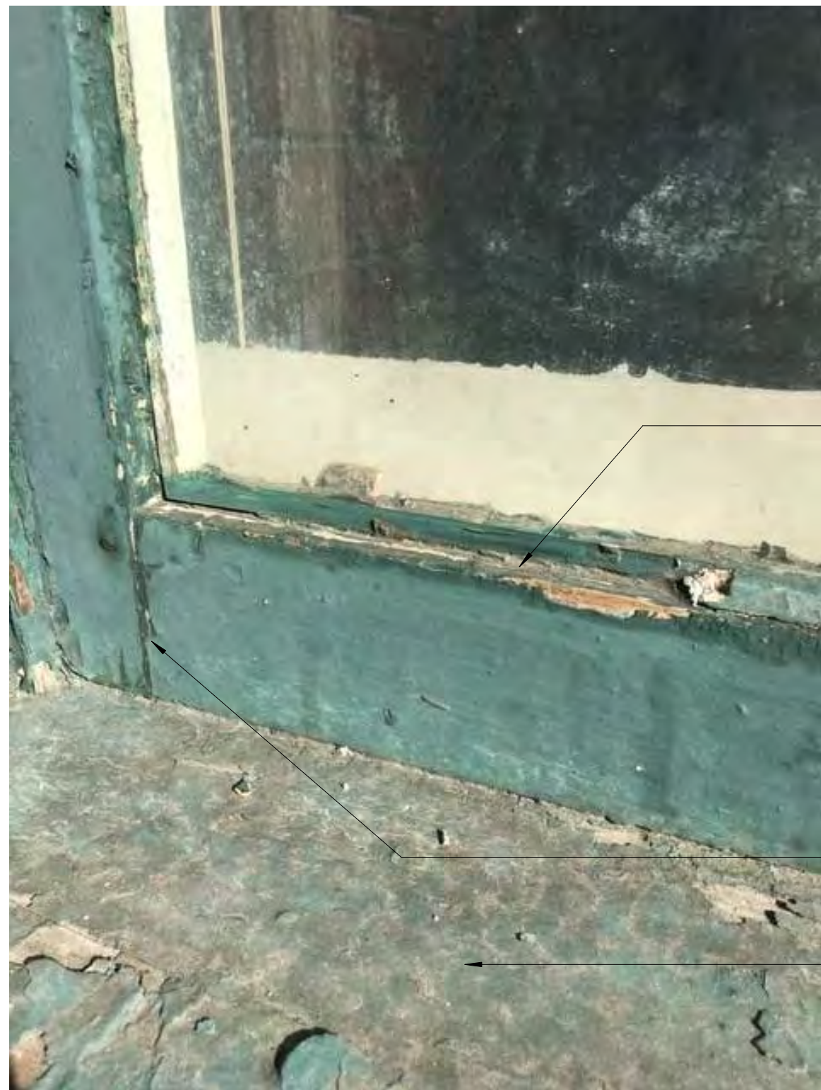
DAMAGED + ROTTING WOOD SHELF
