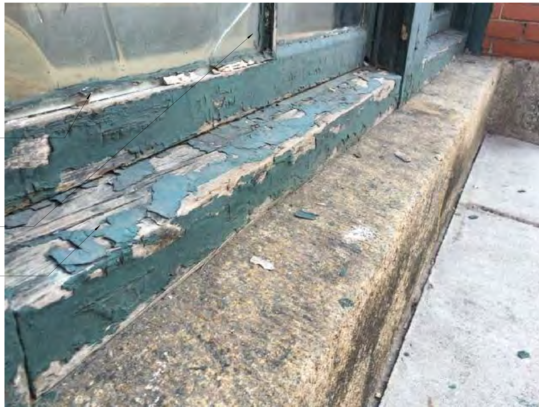
DAMAGED + ROTTING WOOD SILL
