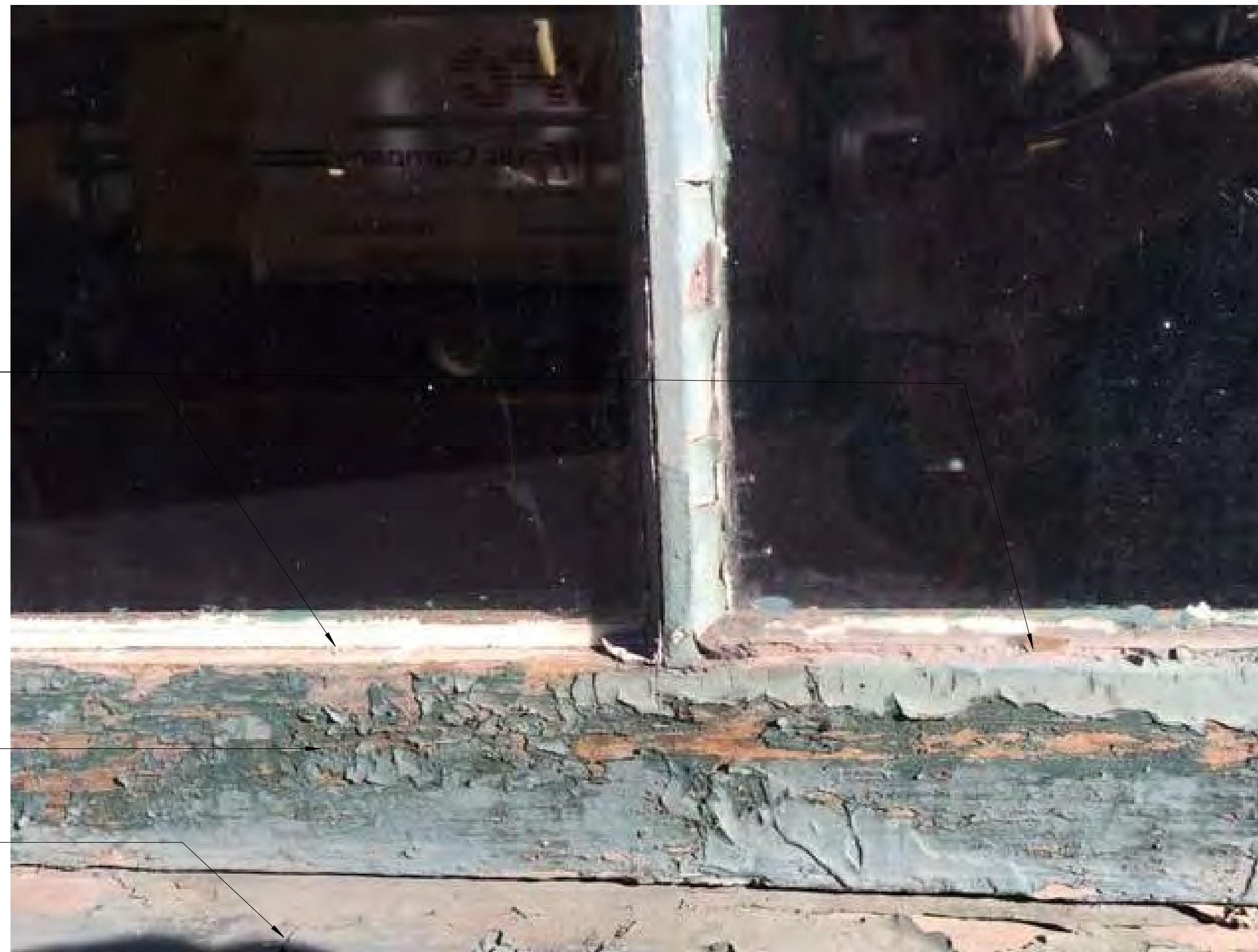
DAMAGED + ROTTING WOOD SHELF
