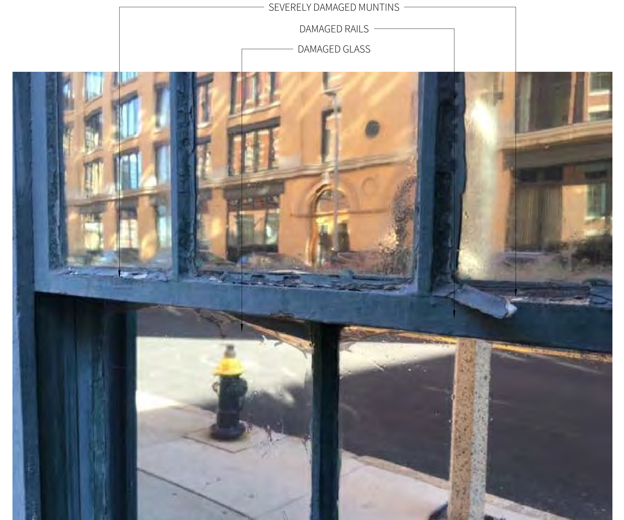
SEVERELY DAMAGED MUNTINS
