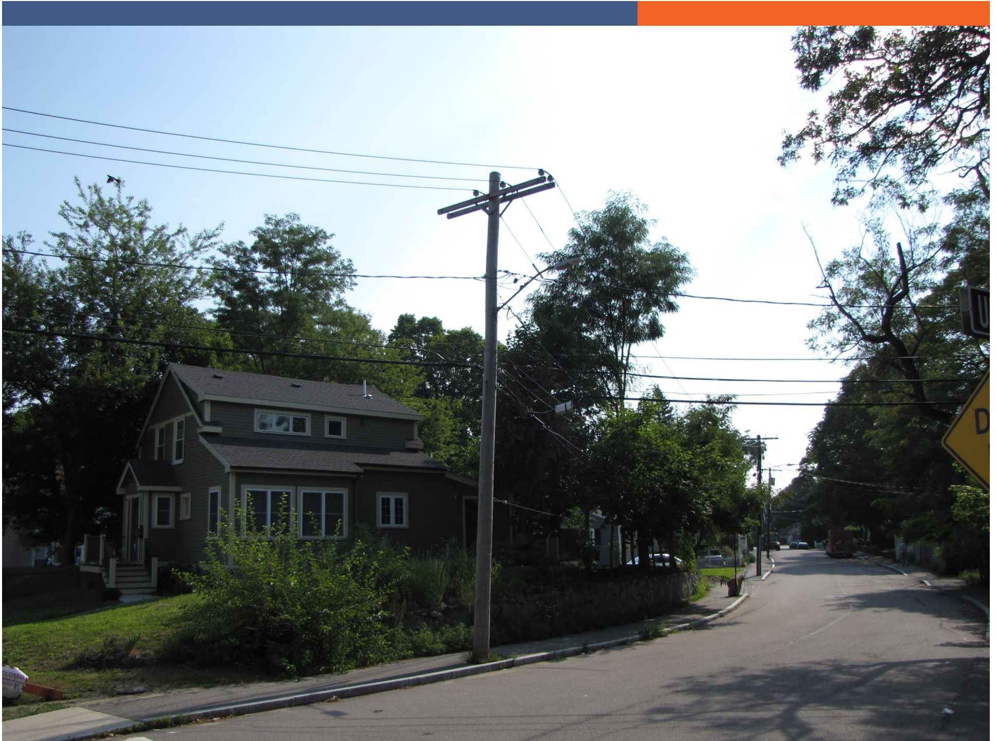
Existing Conditions: Wood utility pole.
