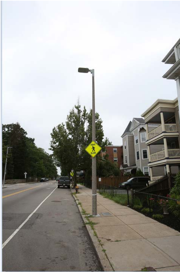
Hex Pole with Aerieta (existing)
