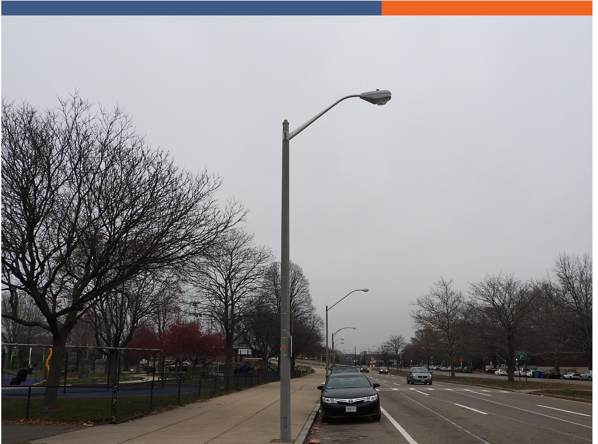
Existing Conditions: Standard concrete light pole.
