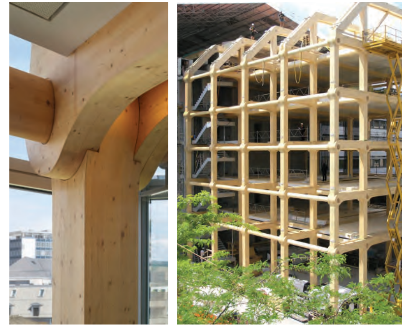
TAMEDIA HEADQUARTERS, ZURICH, SWITZERLAND
